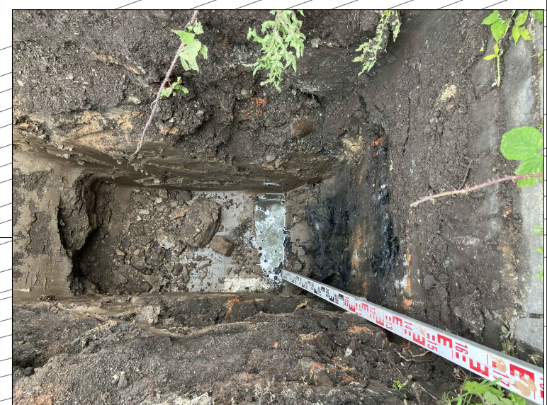
CONCRETE FOOTING ENCOUNTERED AT 1.70mbgl EXTENDING 0.60m FROM VIADUCT FACE
