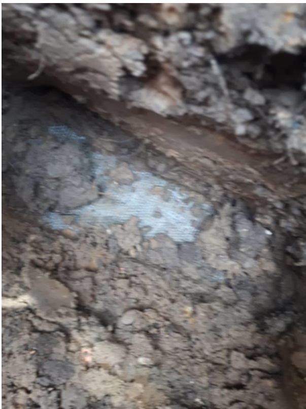
Photograph 3: Plot 197 Geotextile at the base of Validation Pit Location 1
