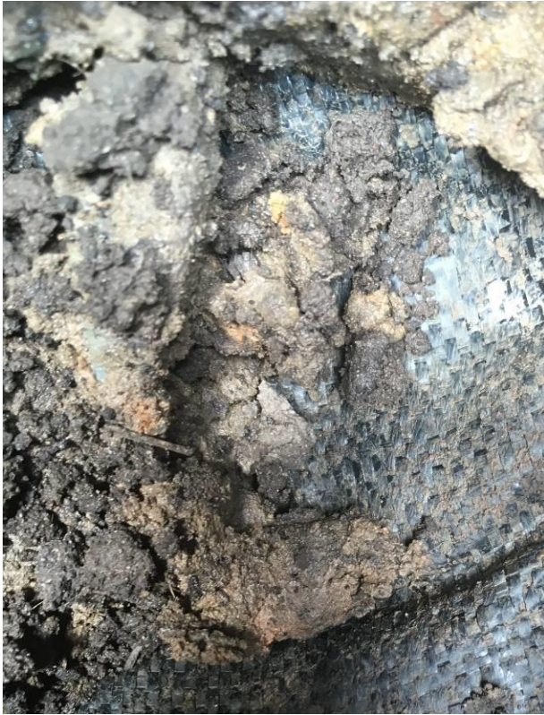
Photograph 33: Plot 190 Geotextile at base of Validation Pit Location 1
