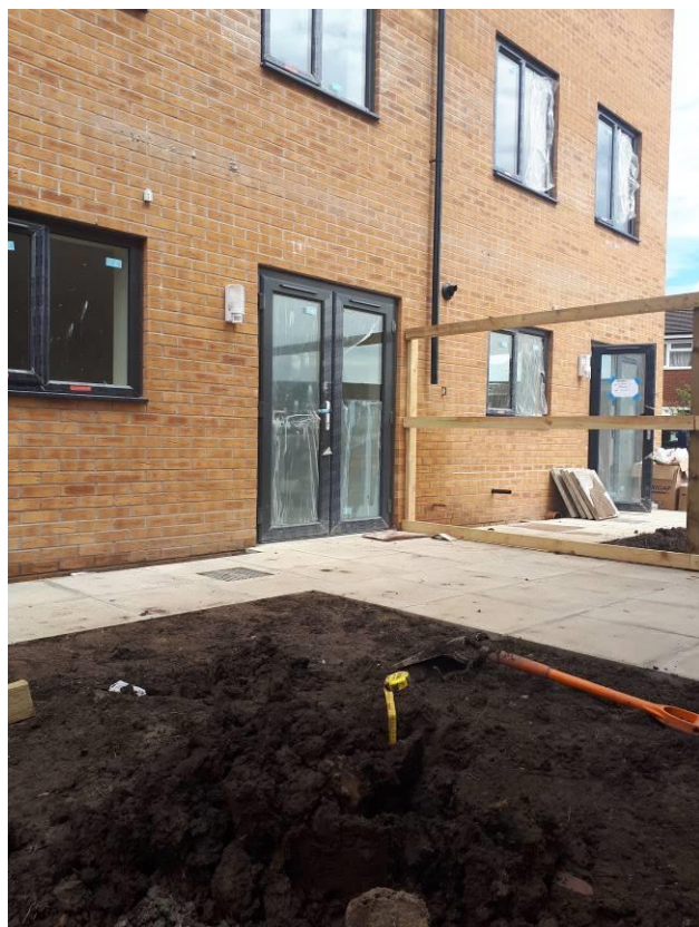
Photograph 7: Plot 198 Validation Pit Location 1
