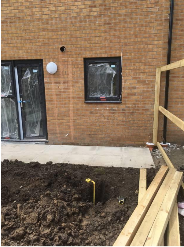
Photograph 25: Plot 189 Validation Pit Location 1
