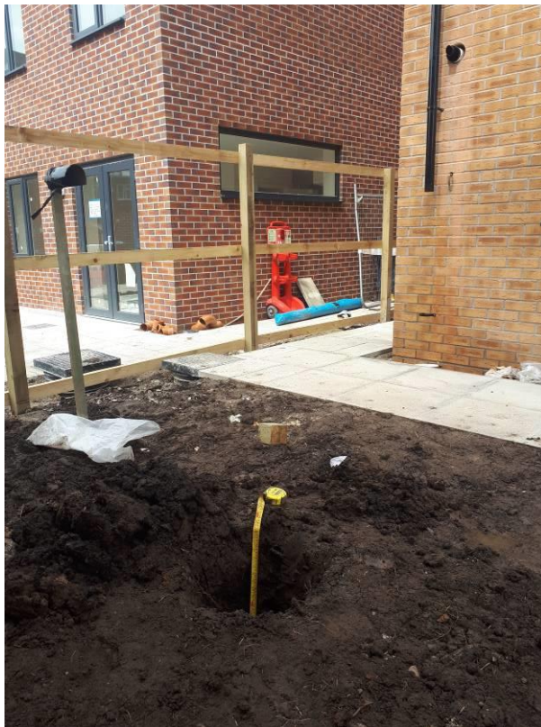
Photograph 10: Plot 198 Validation Pit Location 2
