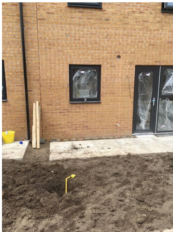
Photograph 58: Plot 194 Validation Pit Location 2
