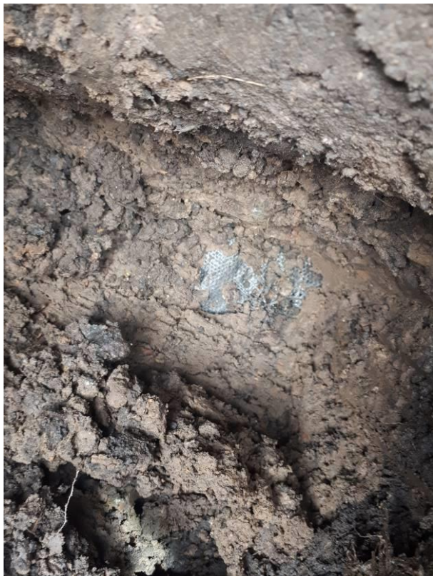
Photograph 9: Plot 198 Geotextile at base of Validation Pit 1
