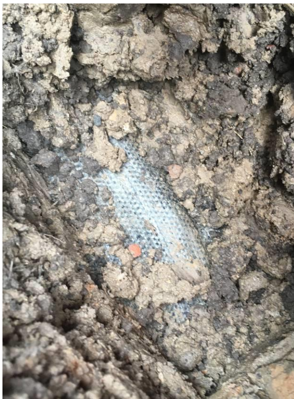
Photograph 60: Plot 194 Geotextile at base of Validation Pit 2
