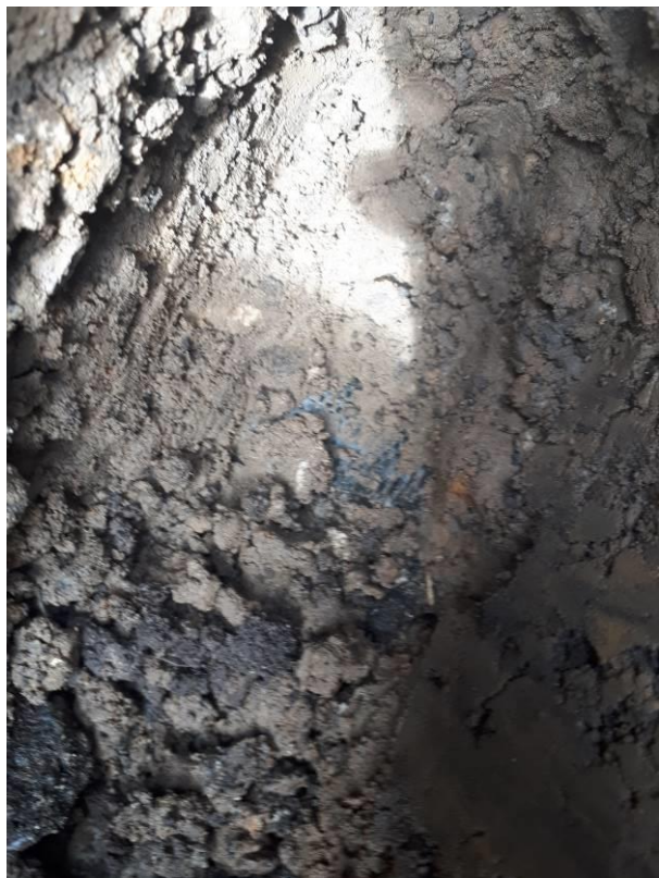
Photograph 15: Plot 187 Geotextile at the base of Validation Pit 1
