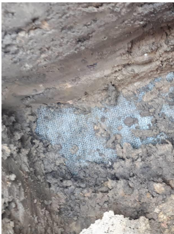
Photograph 57: Plot 194 Geotextile at base of Validation Pit Location 1
