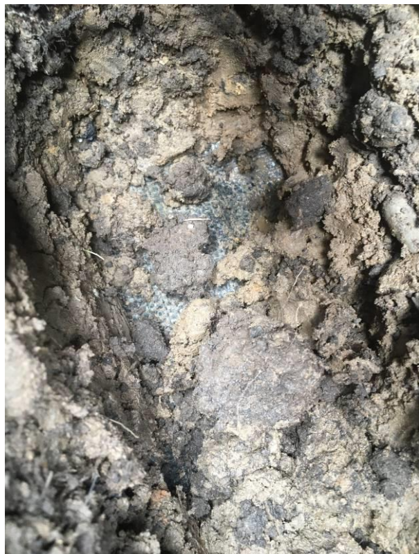
Photograph 36: Plot 190 Geotextile at base of Validation Pit 2
