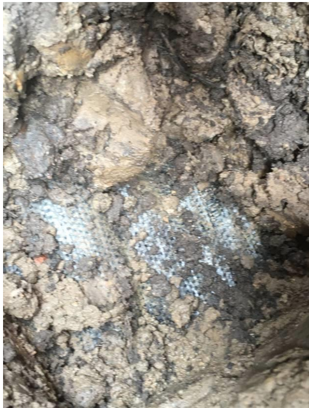
Photograph 48: Plot 192 Geotextile at base of Validation Pit 2
