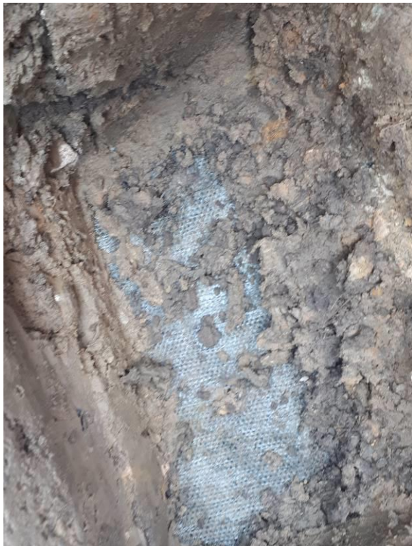
Photograph 39: Plot 191 Geotextile at base of Validation Pit Location 1
