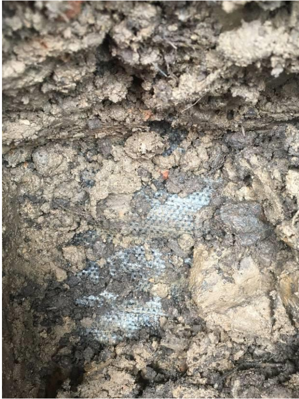
Photograph 45: Plot 192 Geotextile at base of Validation Pit Location 1
