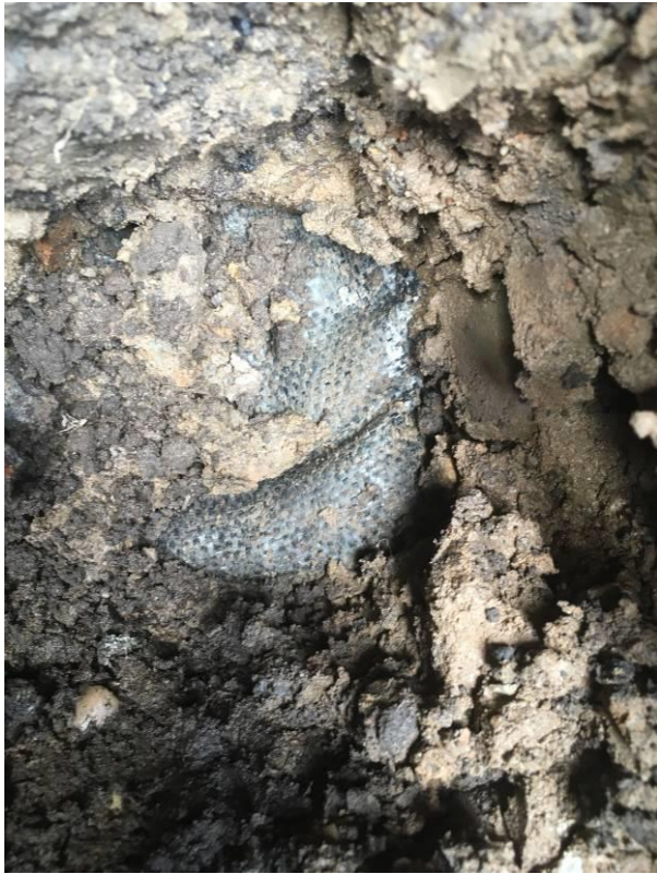
Photograph 21: Plot 188 Geotextile at base of Validation Pit Location 1
