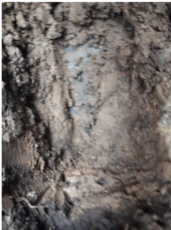
Photograph 12: Plot 198 Geotextile at base of Validation Pit 2
