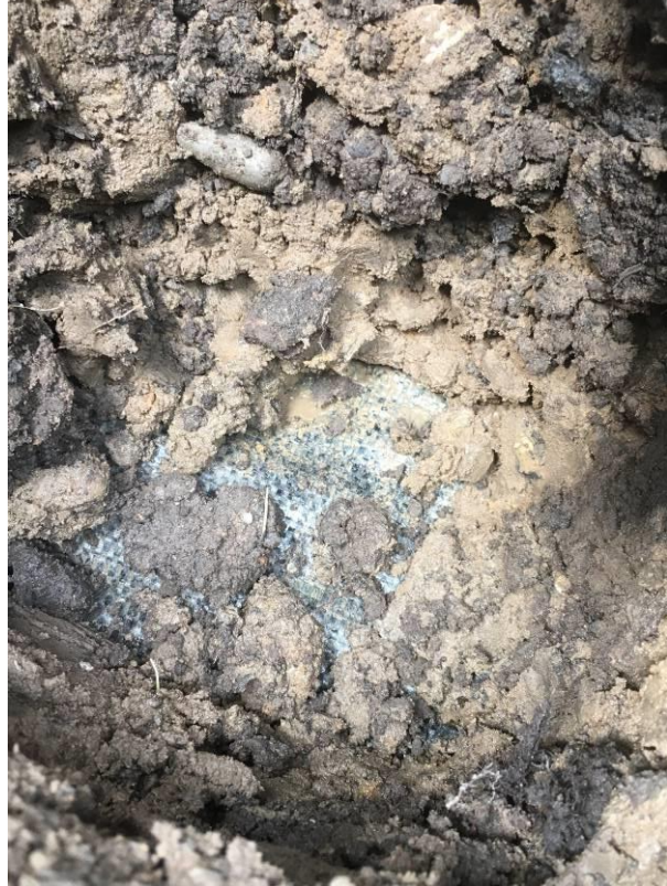
Photograph 54: Plot 193 Geotextile at base of Validation Pit Location 2
