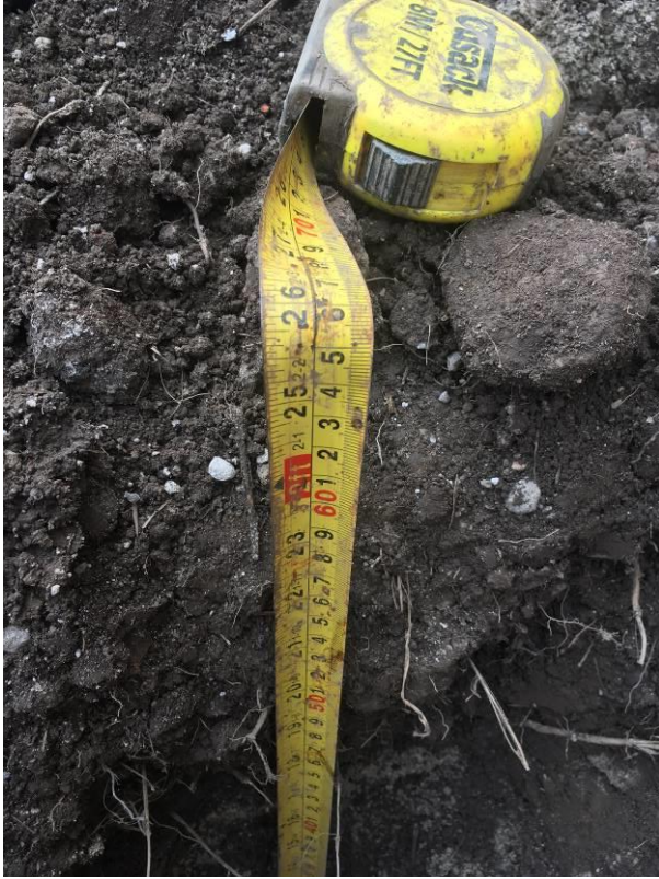
Photograph 53: Plot 193 Validation Pit Depth
