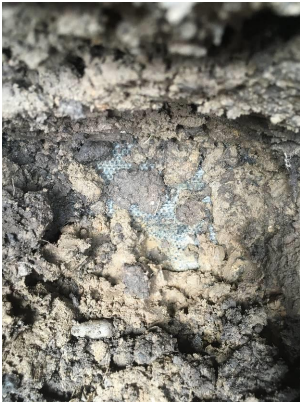
Photograph 27: Plot 189 Geotextile at base of Validation Pit Location 1
