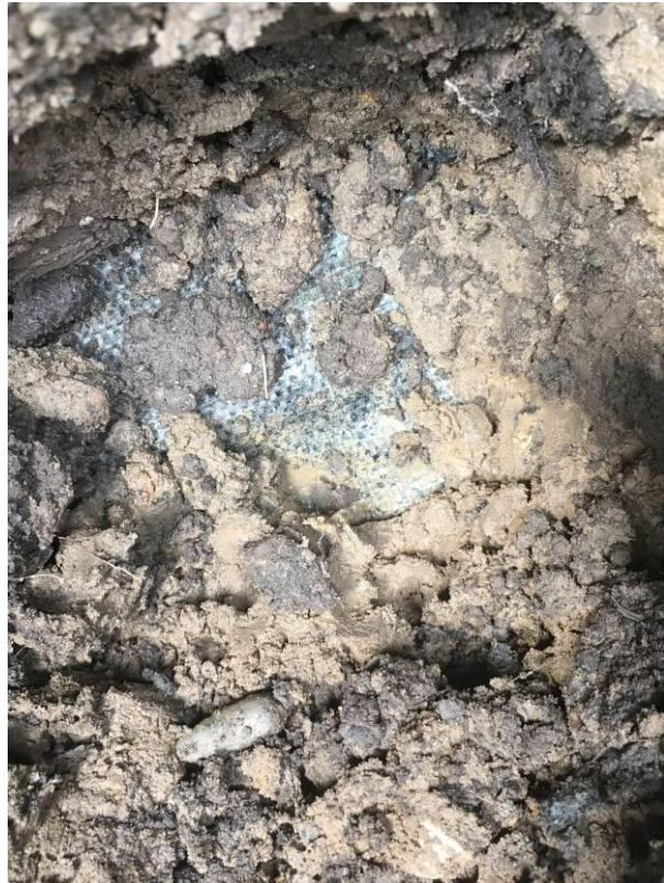
Photograph 42: Plot 191 Geotextile at base of Validation Pit Location 2
