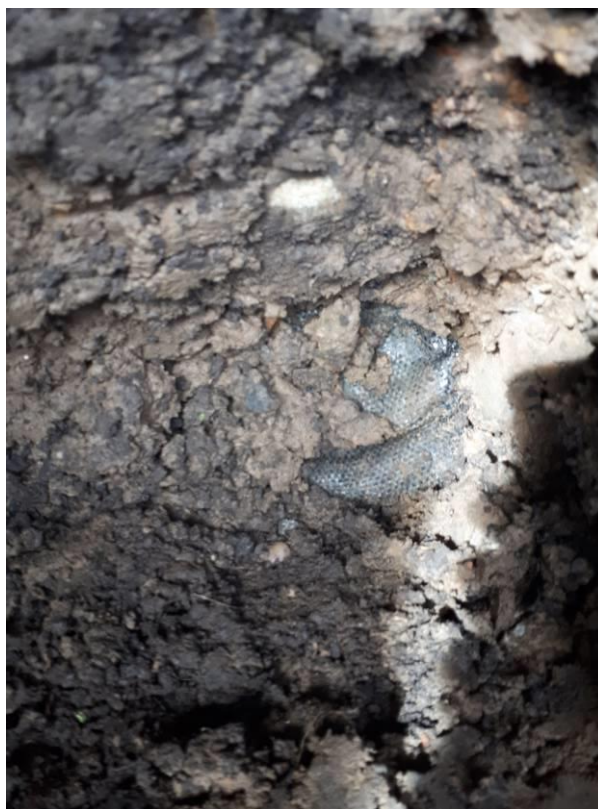
Photograph 18: Plot 187 Geotextile at base of Validation Pit Location 2
