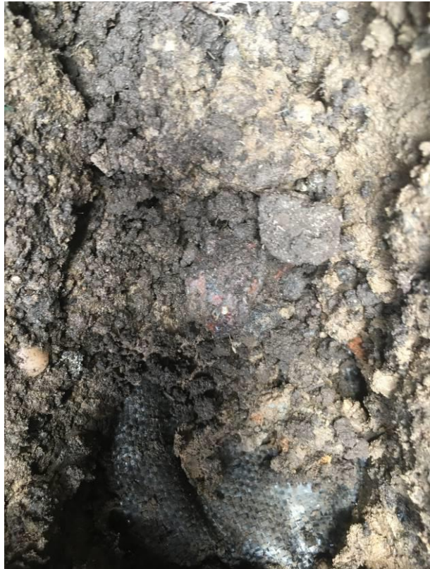
Photograph 30: Plot 189 Geotextile at base of Validation Pit Location 2
