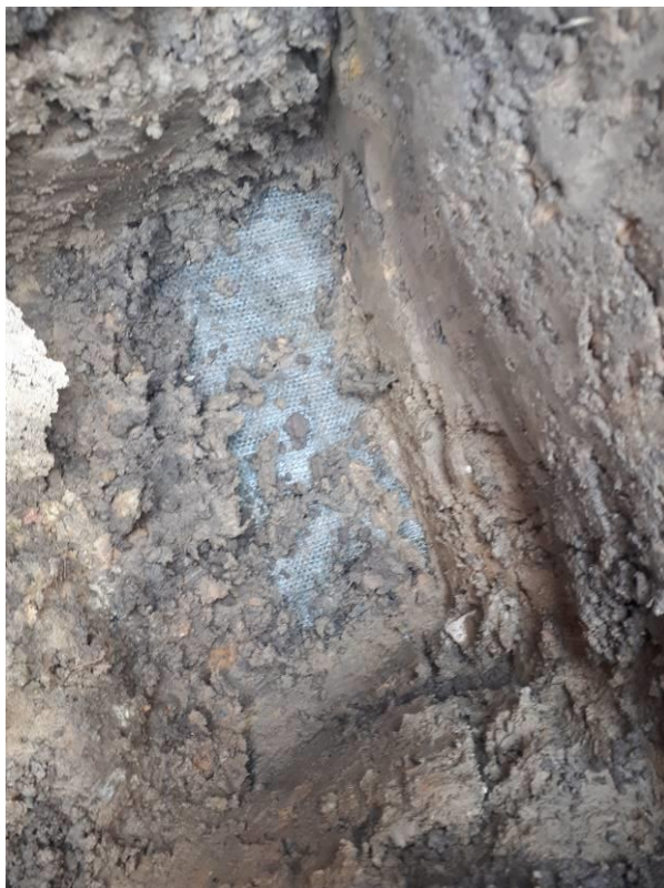
Photograph 6: Plot 197 Geotextile at base of Validation Pit Location 2
