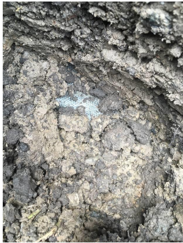
Photograph 24: Plot 188 Geotextile at base of Validation Pit 2
