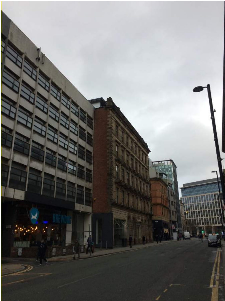
Figure 14 – View along Peter Street towards the east with 37 Peter Street / Freetrade Exchange on the left and the Freetrade Hall to the left. Additionally, no. 47 Peter Street and the Theatre Royal are opposite.
