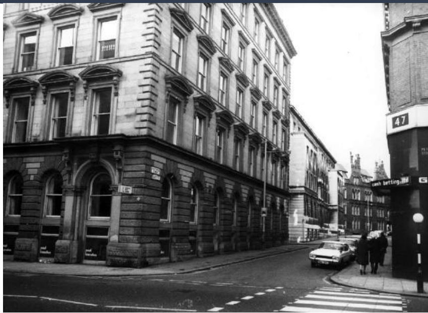
Figure 11: 1974 Historic Image. This image partially shows the Peter Street and Southmill street elevations of 37 Peter Street looking north up Southmill Street. The image shows how the eastern entrance has been altered to install a window to match the other windows along the elevation.
