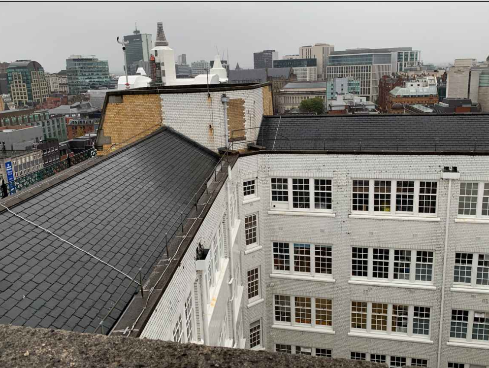
ROOF VIEWPOINTS INDICATING ACCESS ROUTE WITH EXISTING MAN-SAFE RAILINGS
