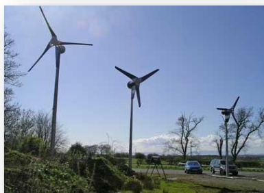
Wind Turbine Installation
