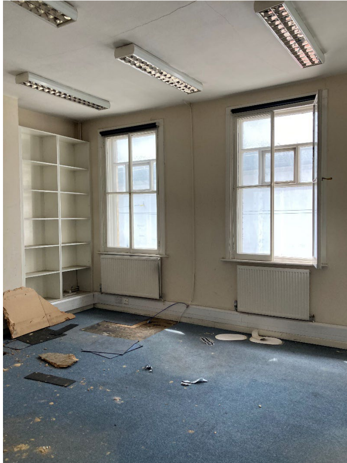
Figure 14: First floor room, looking towards the front elevation, June 2022.
