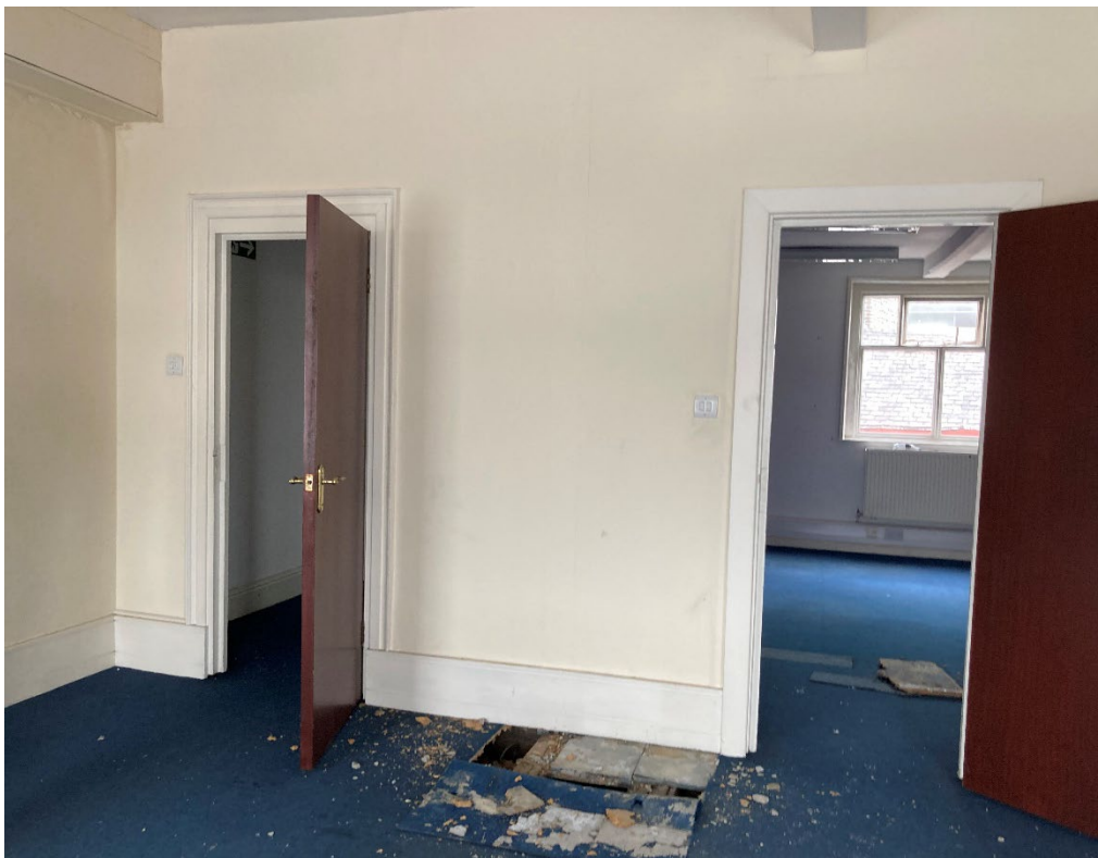
Figure 16: Internal partition between front and back room on the second floor, June 2022.
