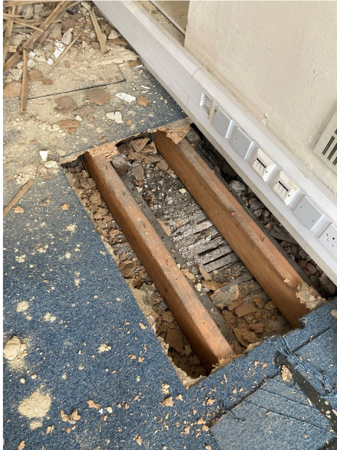
Figure 15: Investigative works undertaken on first floor, showing replaced joists and historic lath and plaster, June 2022.
