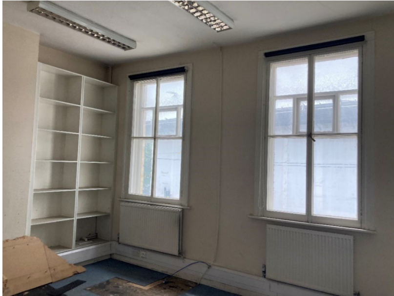
Figure 17: First floor windows with secondary glazing.
