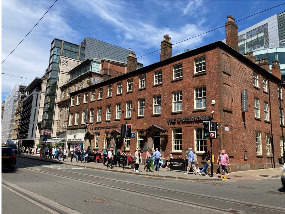
Figure 13: 65 Princess Street- June 2022.
