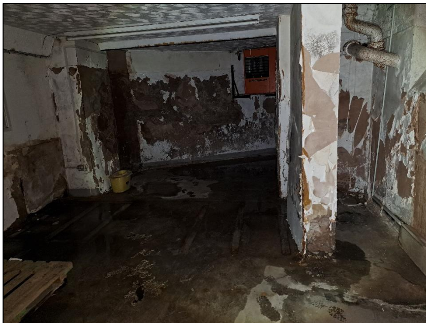
Photograph 12 showing one of the basement rooms
