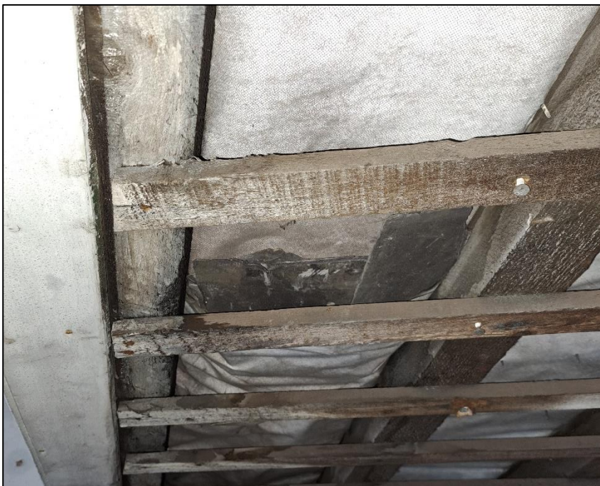
Photograph 7 showing exposed slate tiles
