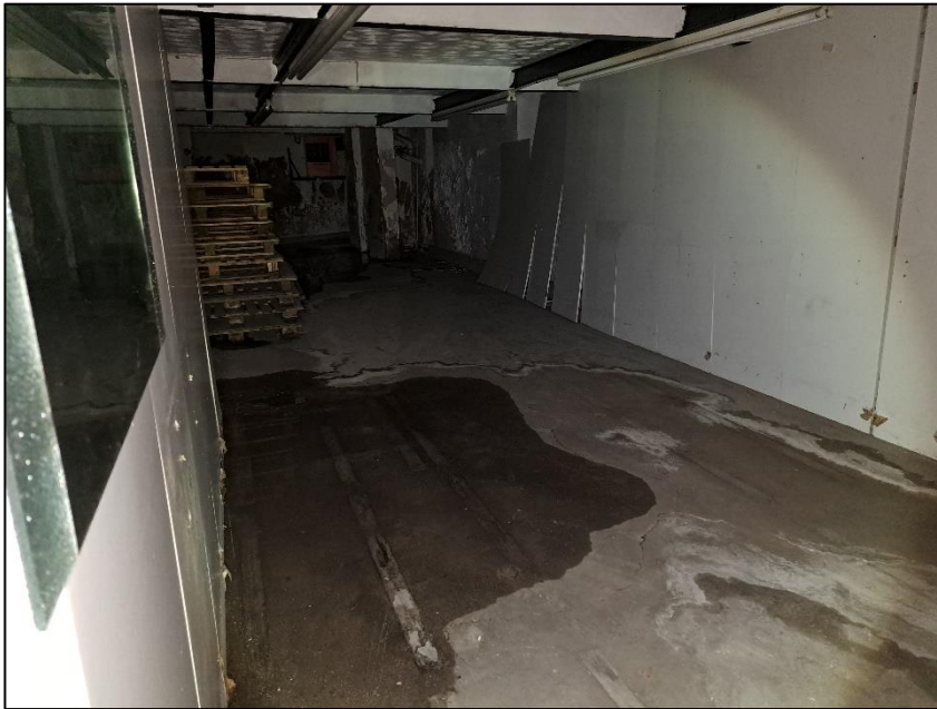
Photograph 11 showing one of the basement rooms
