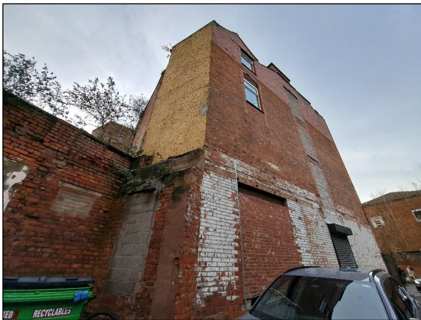
Photograph 3 showing the rear (east) elevation
