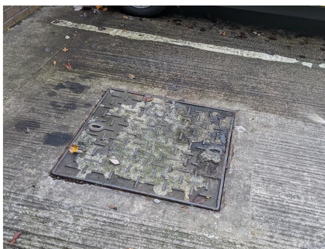
Figure 3 – A manhole cover in the central site section, looking west.
