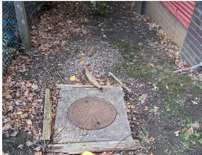
Figure 4 – A manhole located along the southern site boundary on a gentle slope, looking west.
