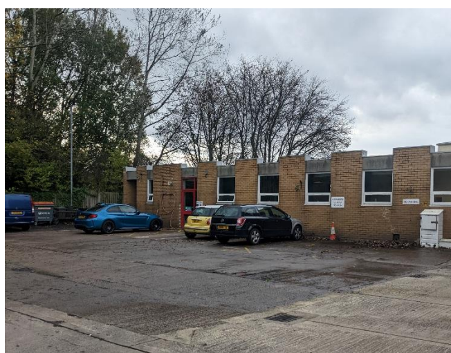
Figure 12 – The central site section with hardstanding and a visitor car park, looking south-east.
