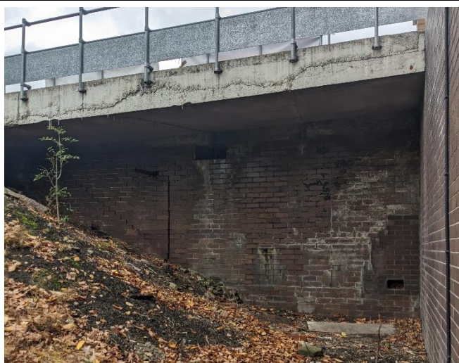
Figure 5 – A retaining wall places across the western slope, near the western site boundary, looking north.
