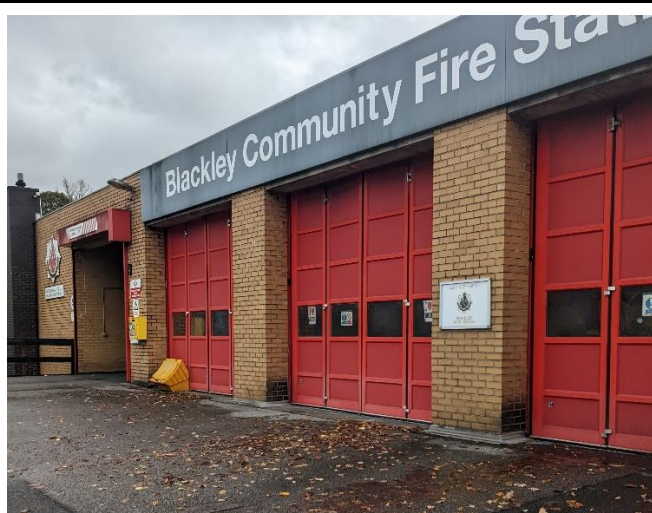
Figure 1 – The front of the Blackley Fire Station with garage entrances, looking north-east.
