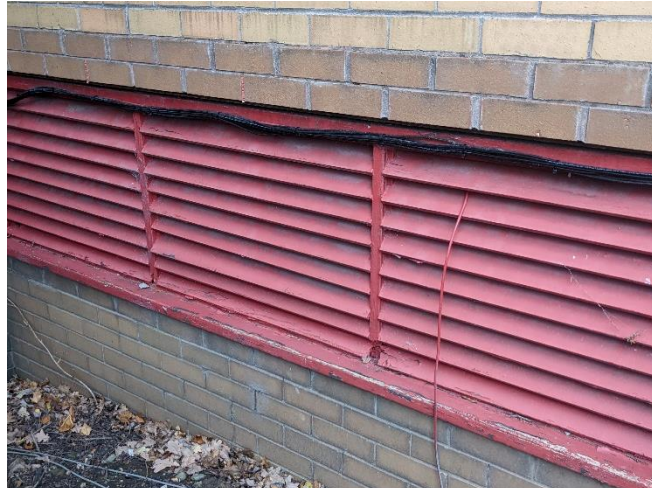
Figure 10 – An electricity substation along the southern fire station building wall, looking north-west.
