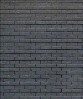
Palmer House - Brick
