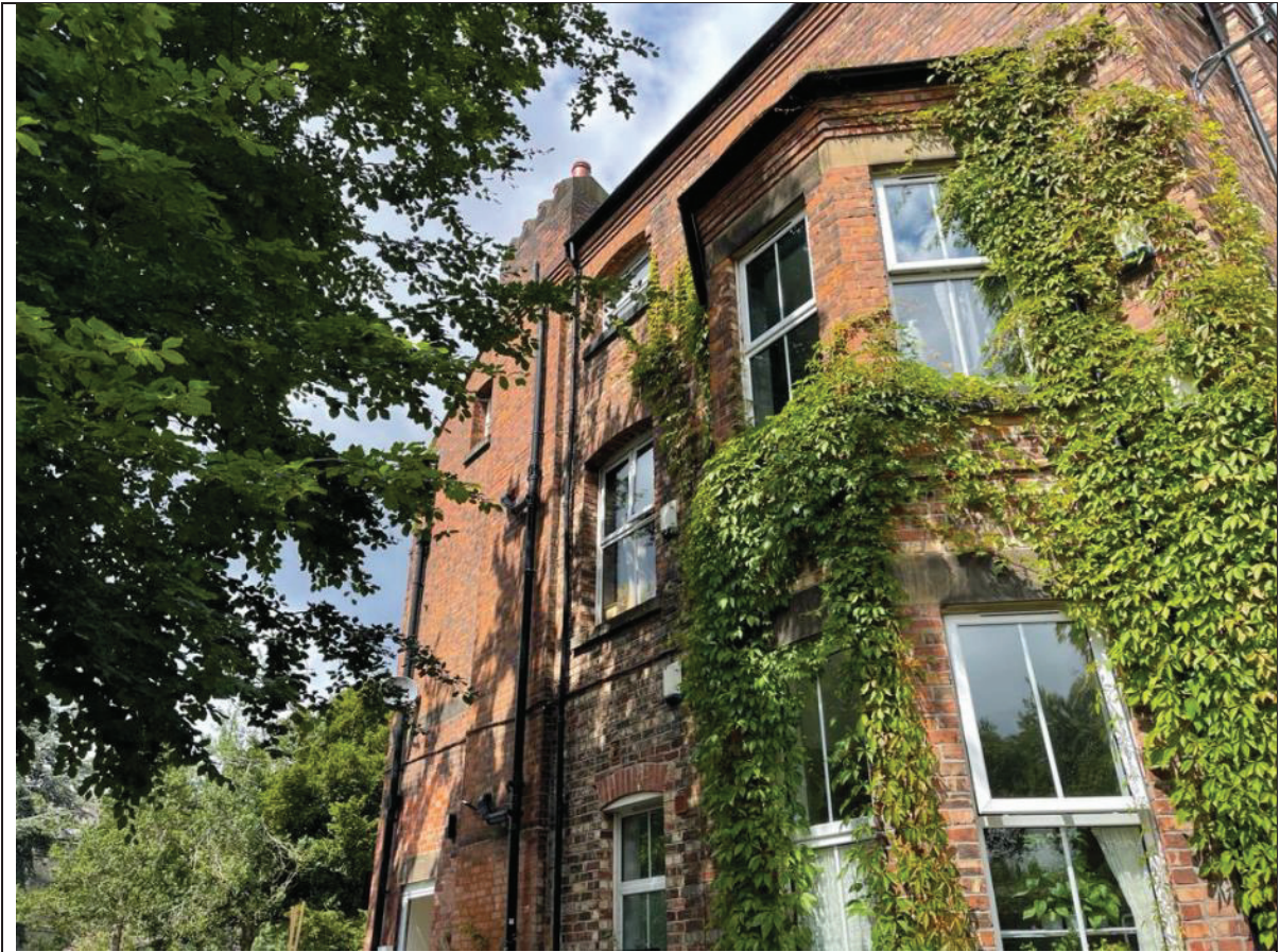
Photo 3: Looking northwards at the southern side of the existing building.
