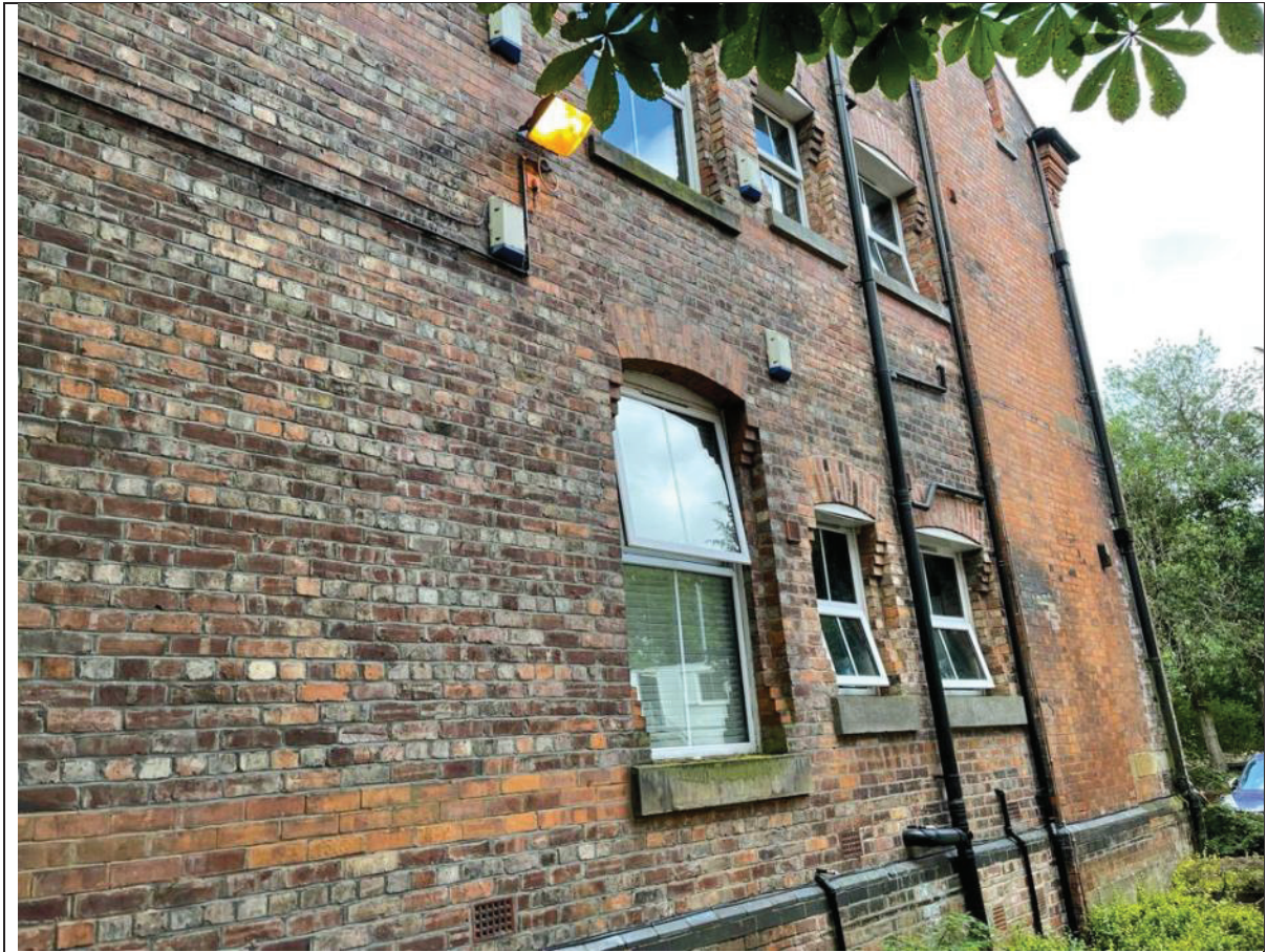
Photo 5: Looking west at the northern side of the existing building.
