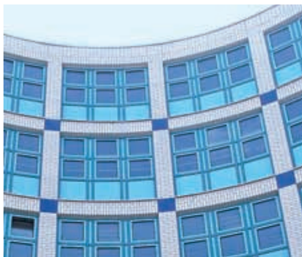
Fig. 21 » ... and spandrel panels
