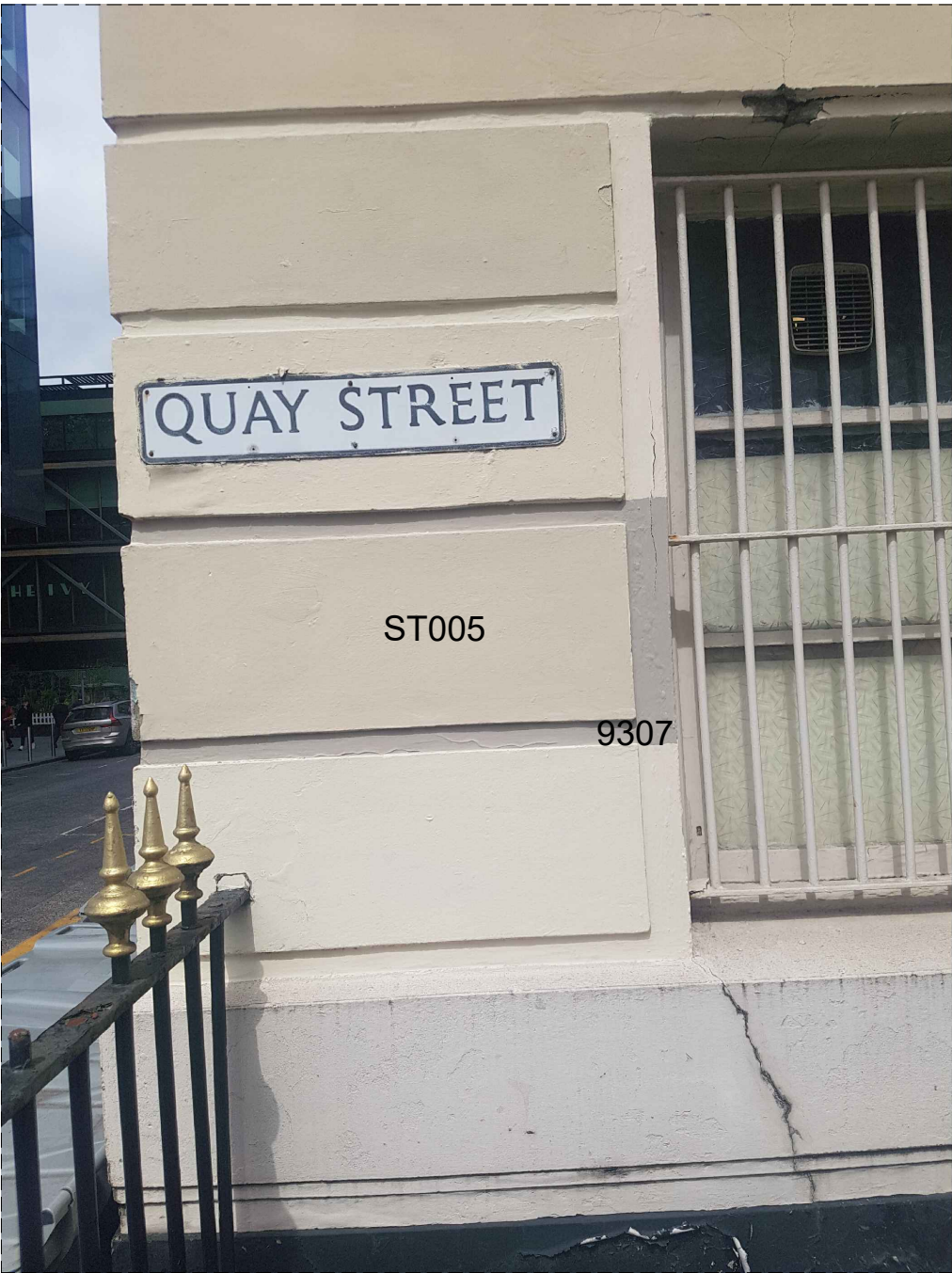
Paint samples for ST005 and 9307 as presented on front corner of the Opera House
