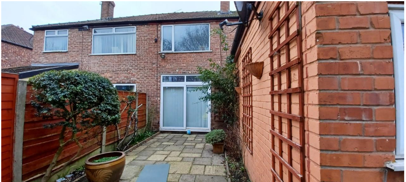
Figure 2. Rear view of the property.
