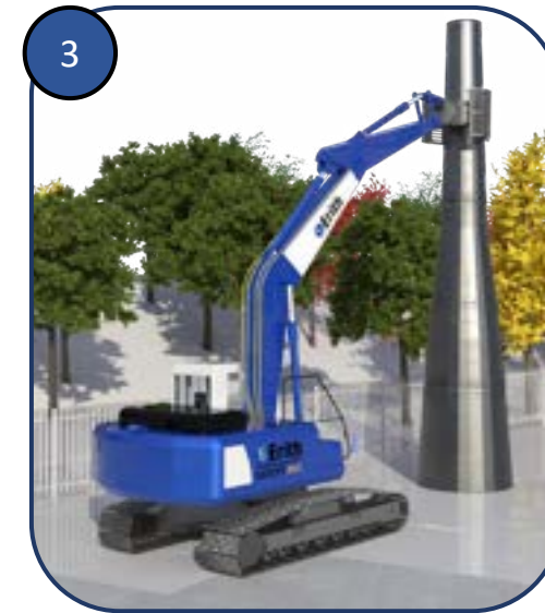
Boiler House & Chimney
