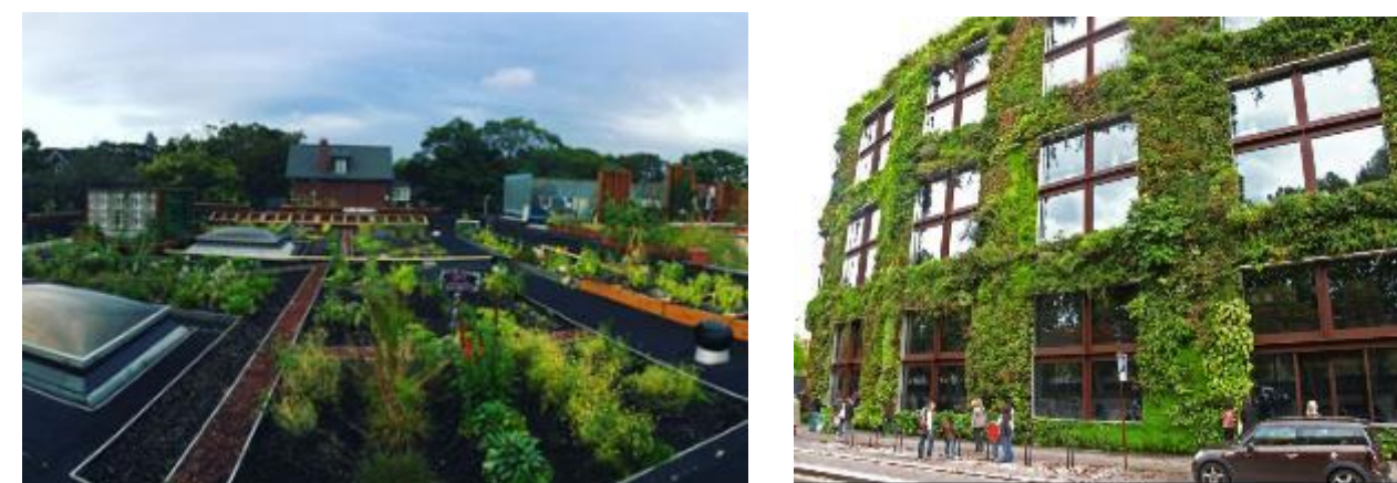
Figure 10 - Green roofs and green walls
