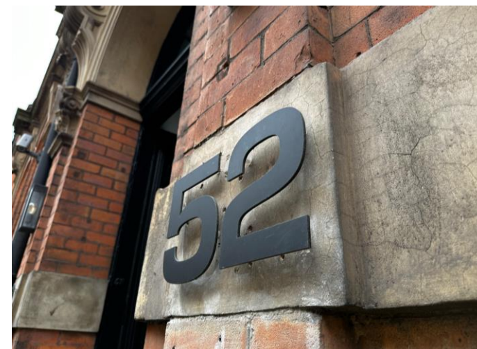
Existing building signage, 52 Princess Street
