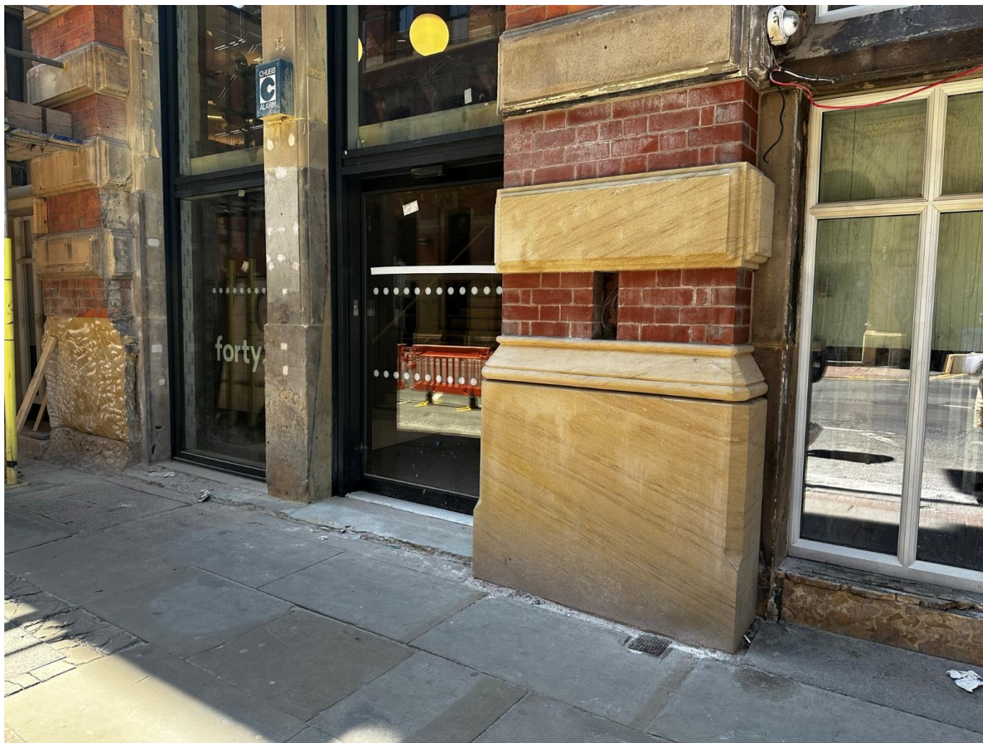
Current photograph taken during construction phase showing new replica stone band, on which the signage is proposed. Below it, new masonry courses and a new stone plinth.
