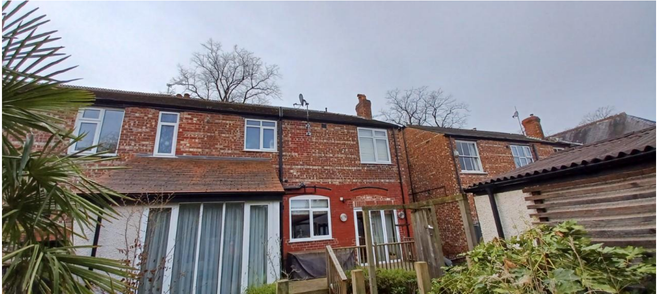
Figure 2. Rear view of property.
