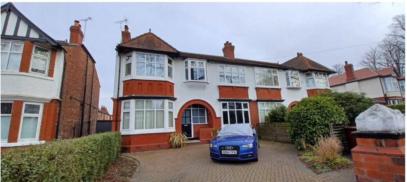
Figure 1. Principal elevation of No.22 Darley Avenue.
