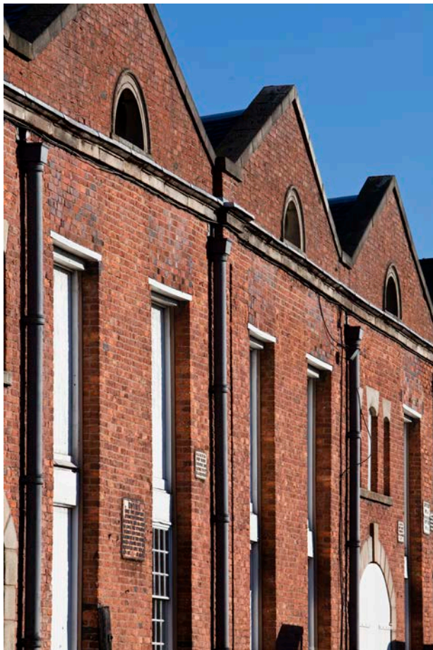
Figure 1: Façade of the 1830 Warehouse, showing rainwater downpipes in situ
