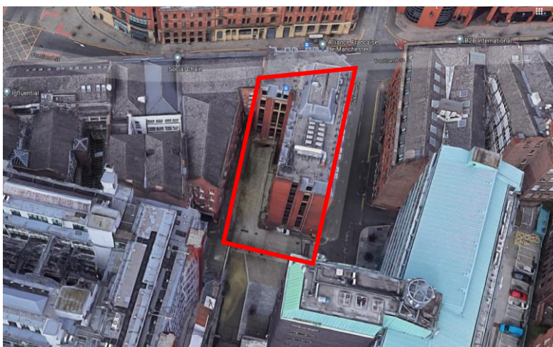
Plate 1 – View from south of rear of building.
