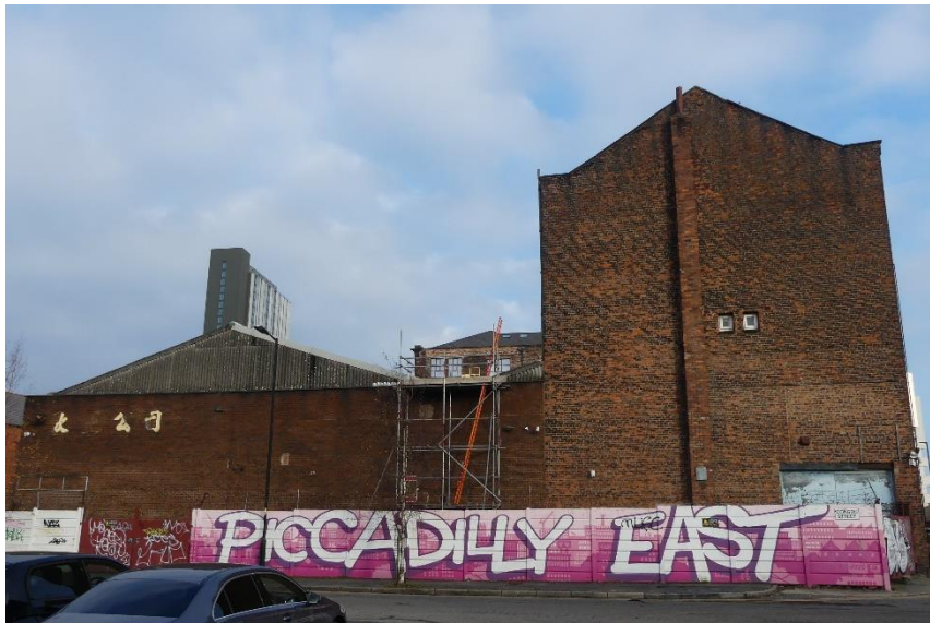
Figure 4.10: The southern elevation of the application site adjoining the single-storey warehouse
