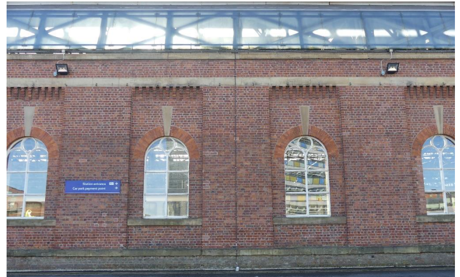
Figure 4.21: Detailing to the northern elevation of the train shed
