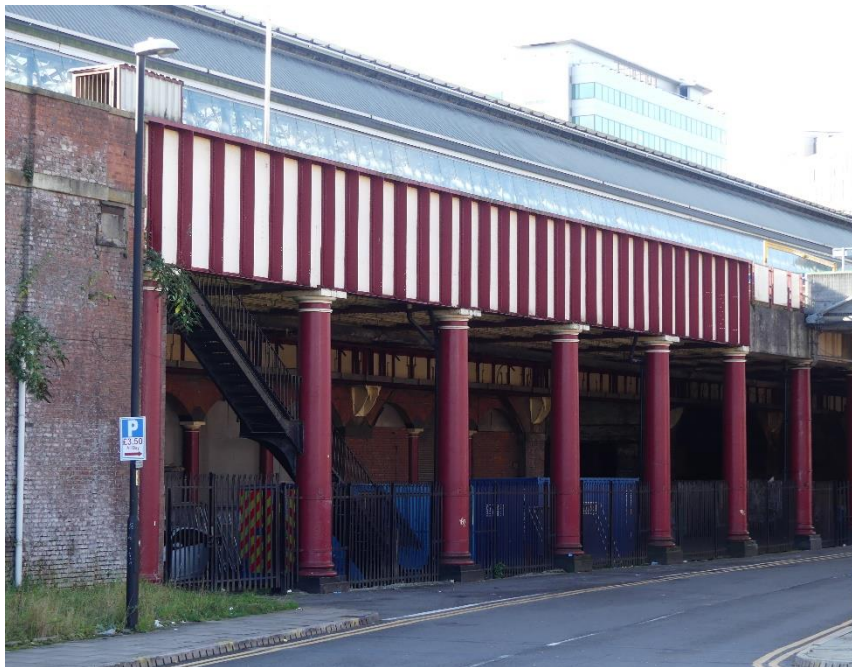
Figure 4.20: Part of the station undercroft
