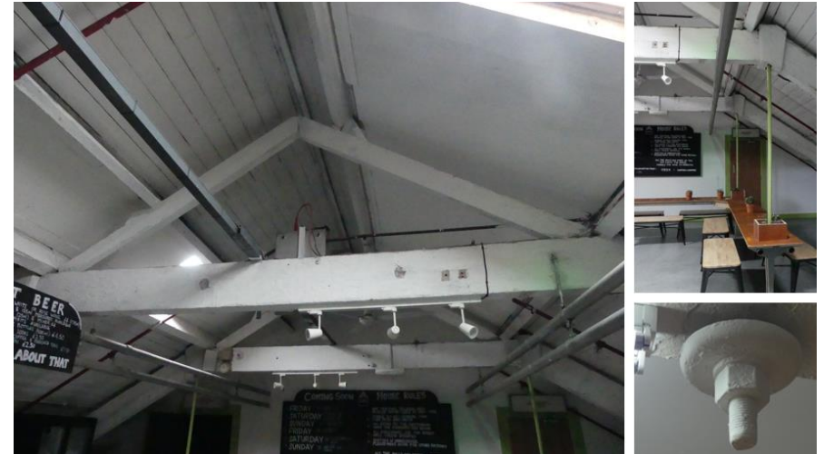
Figure 4.14: The interior of the roof and detail of the tie rods that are fastened through the floor beams
