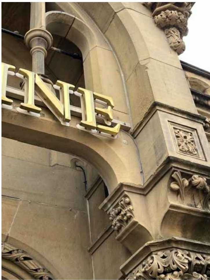
IMAGE 1 - EXISTING SIGNAGE DETAIL AND ELECTRICAL CONNECTION
