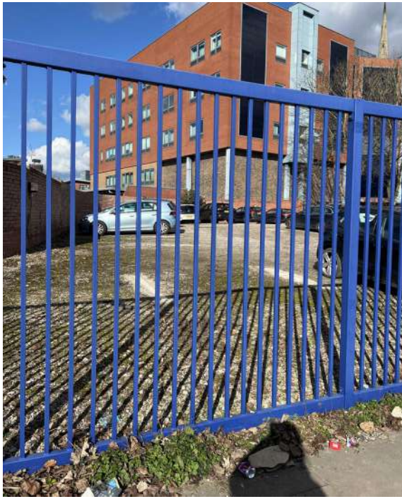
2 - View of existing fence from footpath towards E&K building.
