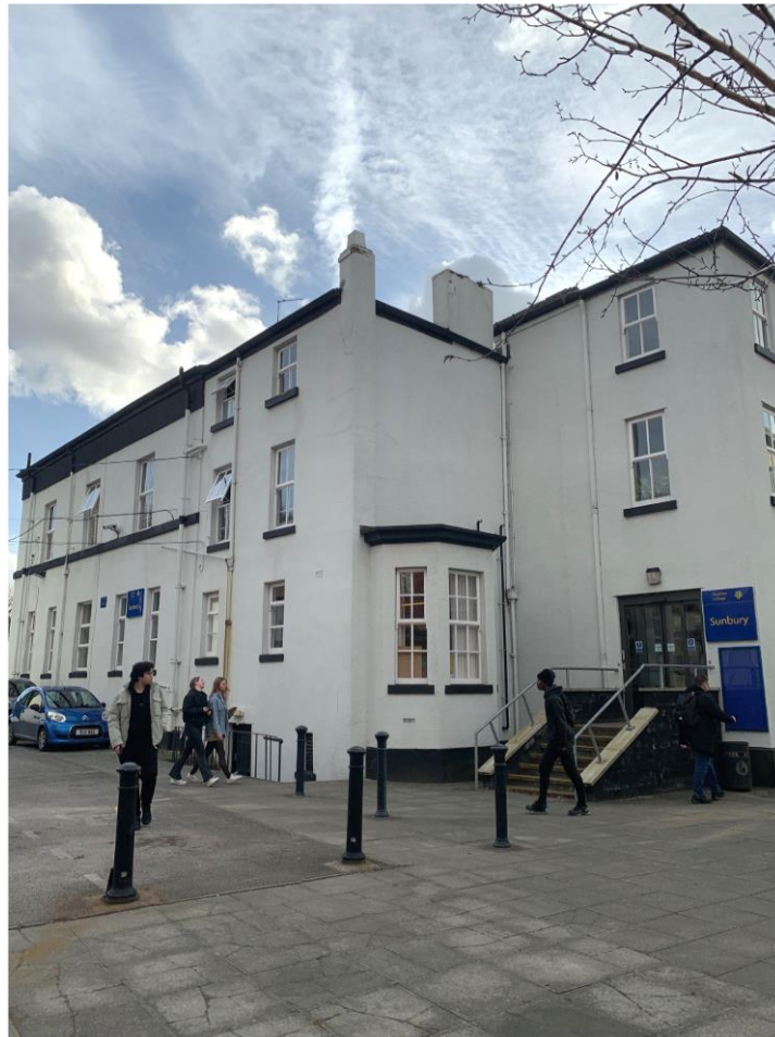
Figure 2 – Existing Building on Site
