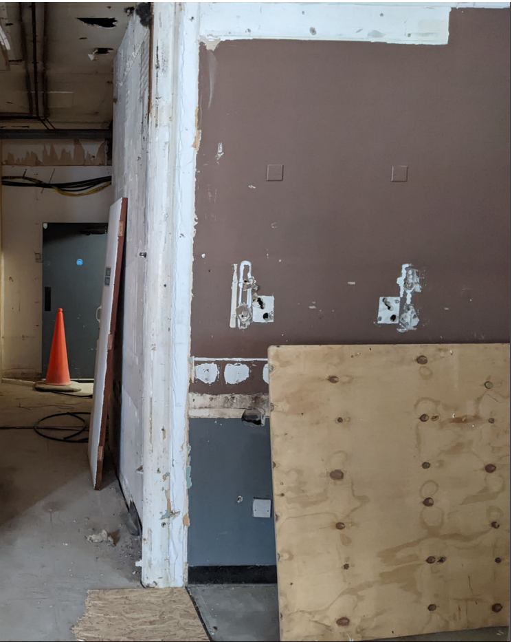
IMAGE SHOWING EXISTING BUT NON-ORIGINAL STUD WALL
