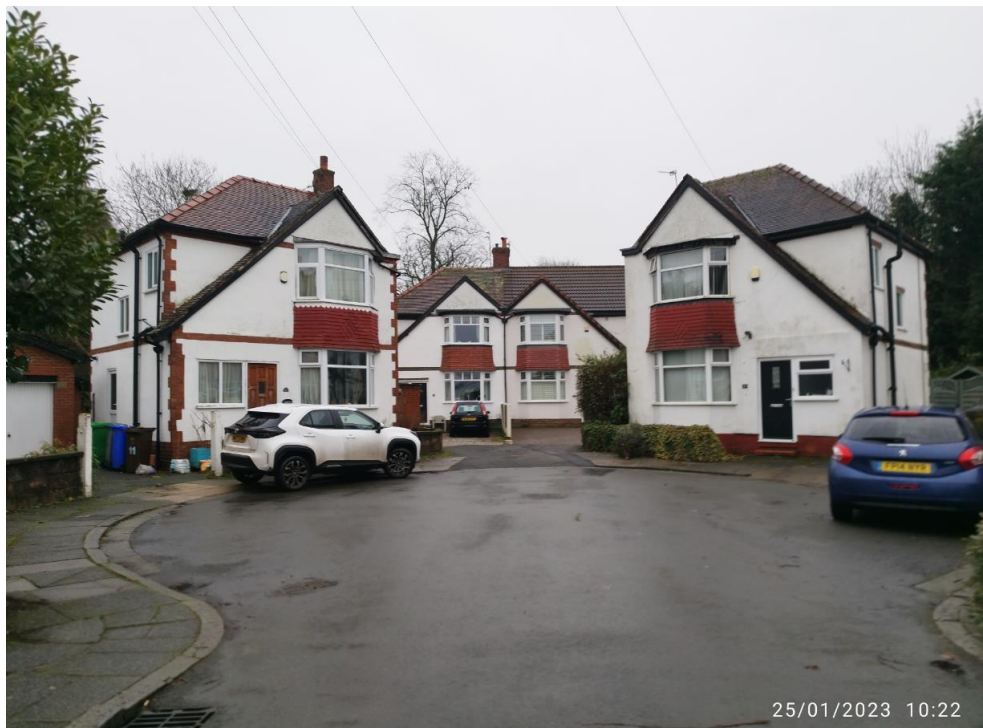
Above image of the two houses at the end of Highcroft Avenue with unusual juxtaposition
