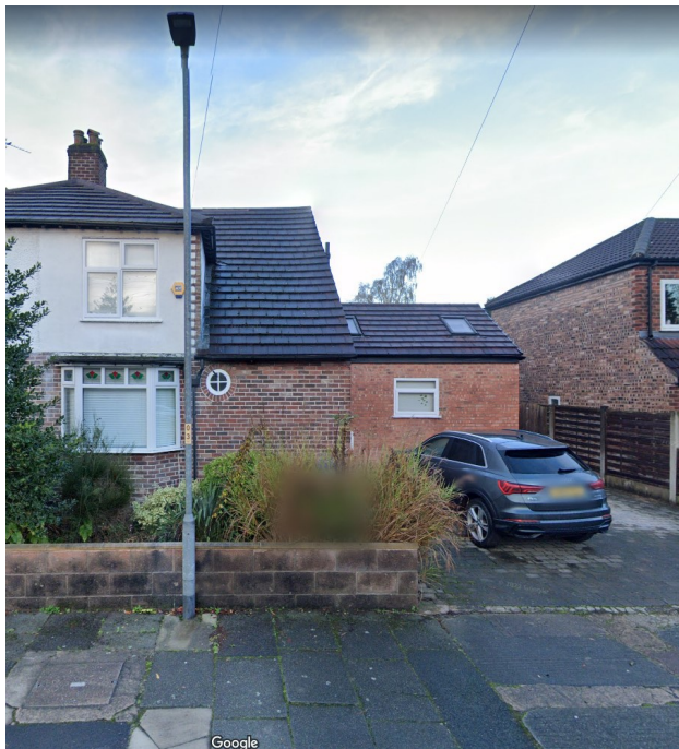
Existing Front elevation showing existing side extension
