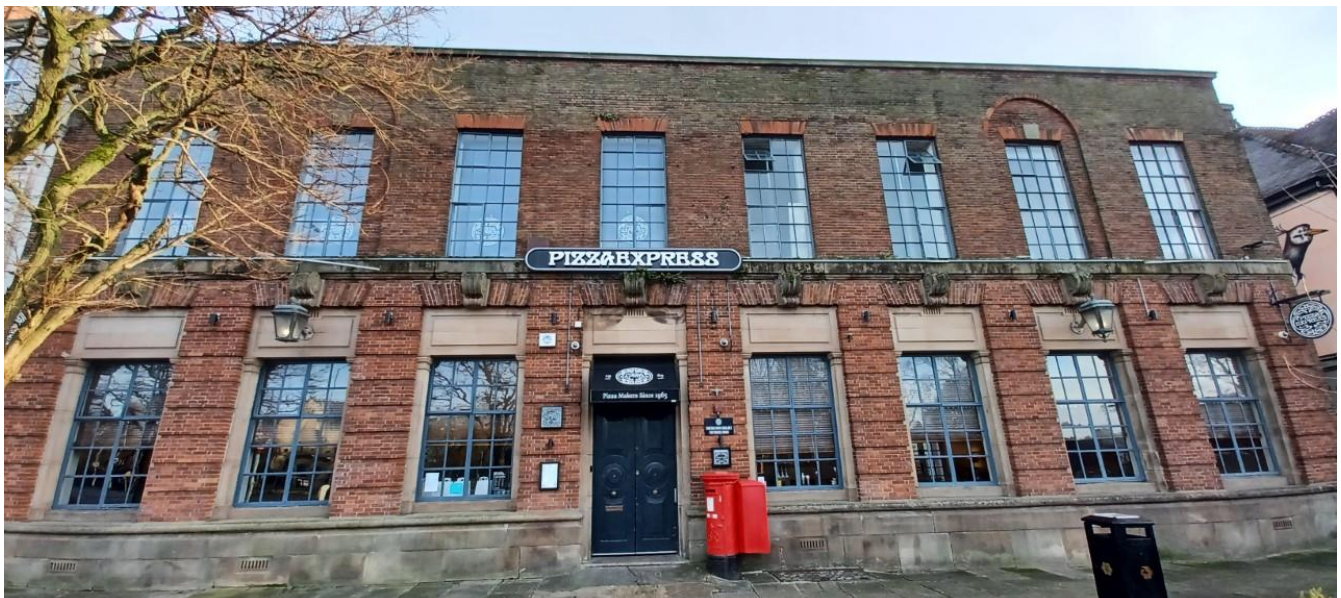
Figure 1. Photograph of the principal elevation of No.95 Lapwing Lane.
