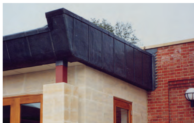
Fig 62. Standing seam
