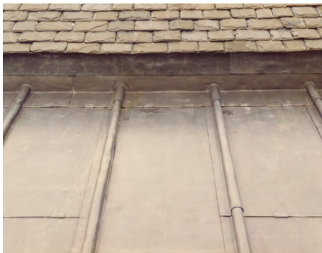
Fig 240. Abutment finishes (30° and above)
