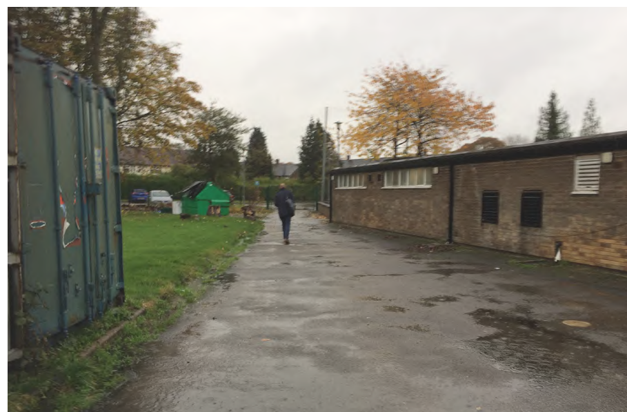
4. Looking onto service road
