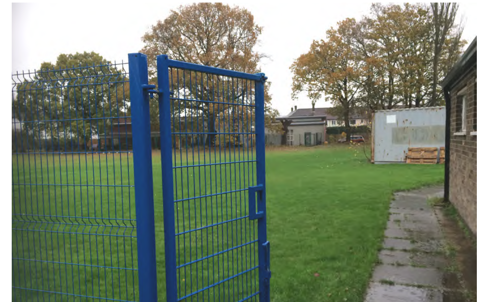
2. Looking towards Sure start and containers
