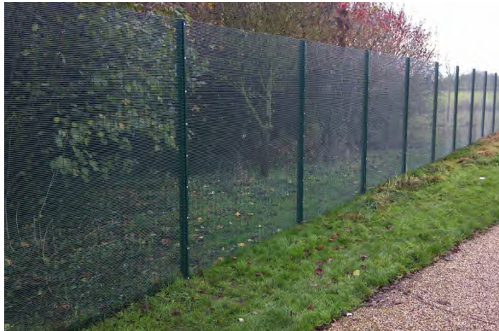
Internal Weld Mesh Fencing (2.4m High)
