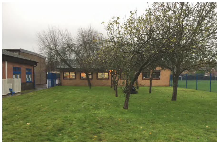
8. Centre of the site - trees adjacent to Block C (EFAC) to be removed
