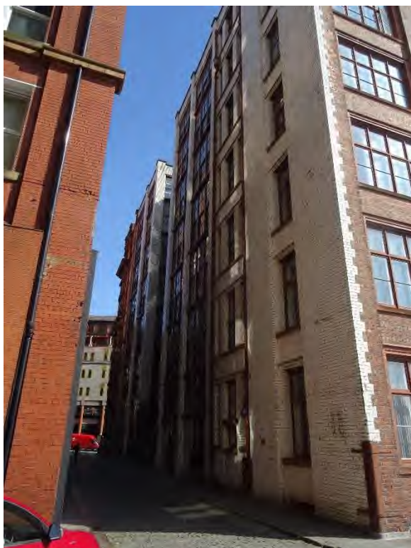
Figure 4.5: Functional side and rear elevations to the narrow warehouse passageways
