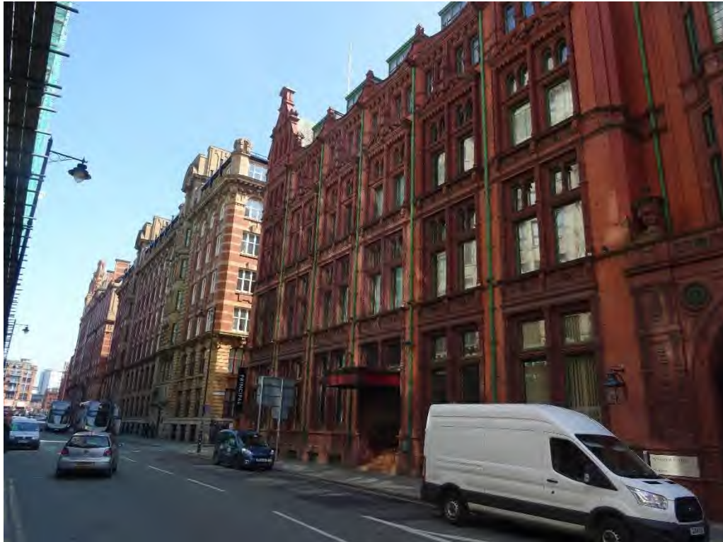
Figure 4.4: The Whitworth Street frontage
