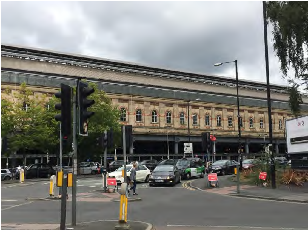
Figure 4.16: Train Shed to Piccadilly Station
