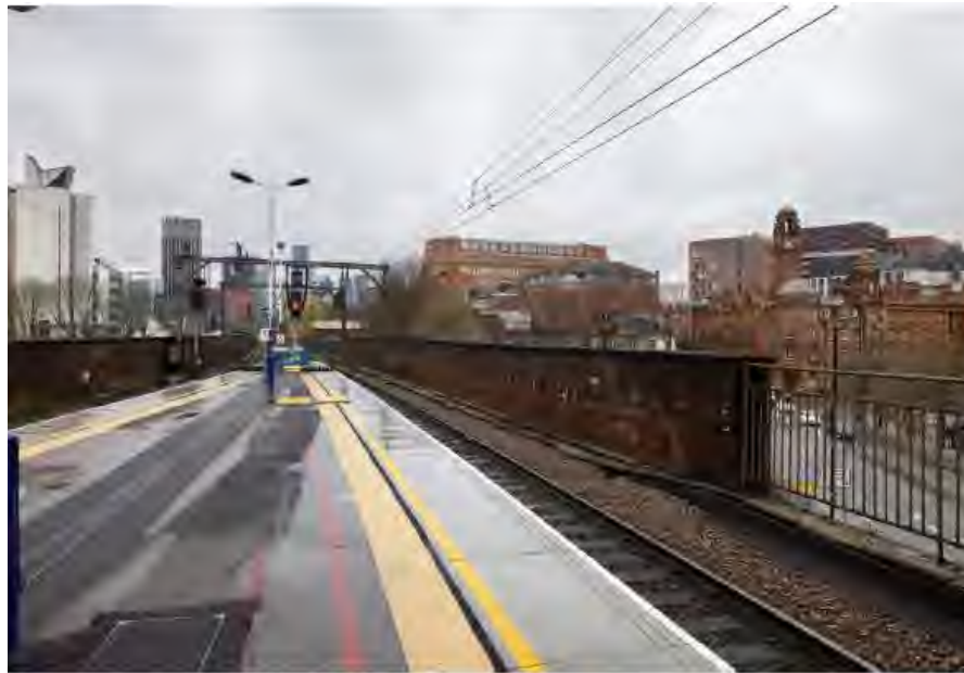
View 3: From Piccadilly Station Platform 13/14 (Existing)
