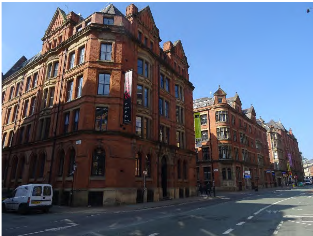
Figure 4.3: The western frontage of Princess Street
