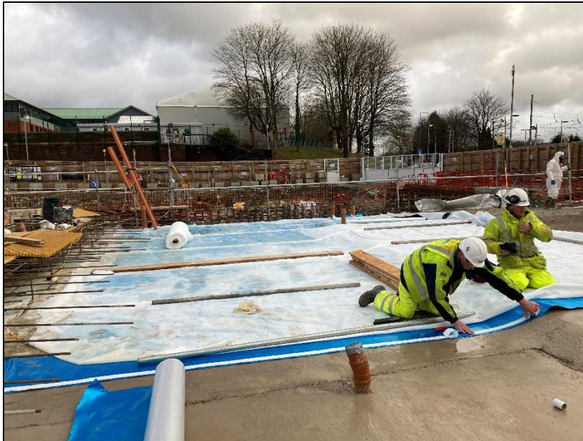
Photograph showing the area with Visqueen Gas Barrier membrane in process of installation in the central upper raft area of the site (dated 14 th February 2022), prior to Ramboll site attendance. Photograph taken facing south-east.
