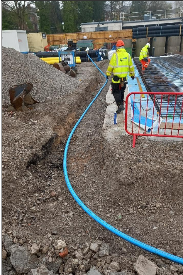
Photograph showing the proposed route for the water barrier pipe, which is adjacent to the building footprint (on the right). The photograph is taken facing the north-east.
