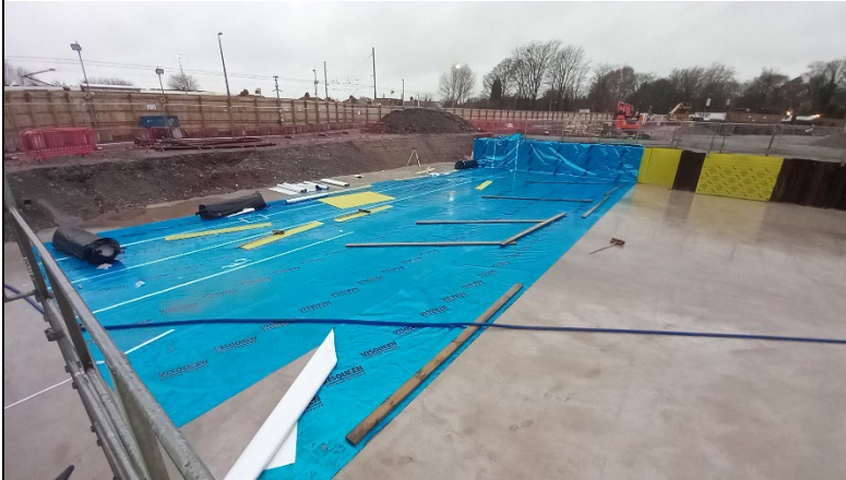
Photograph showing the area with Visqueen Gas Barrier membrane requiring resealing due to the weather. Photograph taken of the Basement Area, facing the west.
