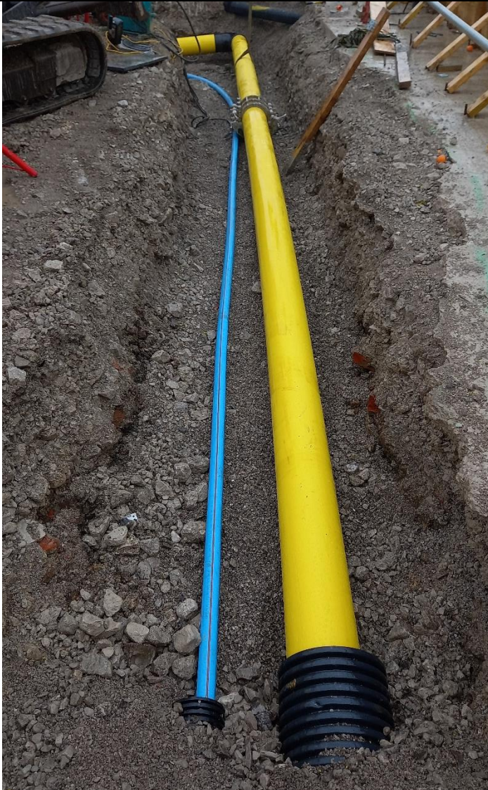
Photograph of the water barrier pipe crossing the site with the building footprint on the right. The route is roughly crossing the site in a north-easterly direction.
