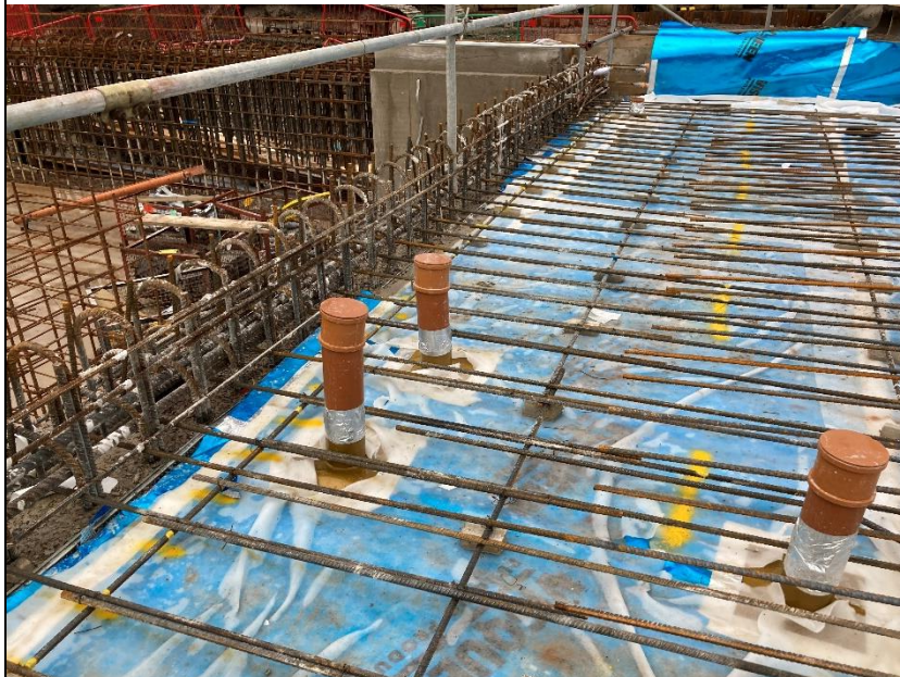
Photograph of a service pipe entry seals around the service ducts in the upper raft area. These were further sealed with GR foil lap tape
