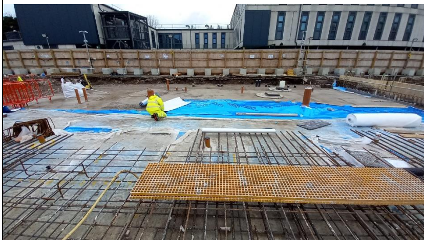
Photograph of the membrane installation underway towards the north-eastern site boundary. The membrane is laid down in strips. Photograph taken facing the north-east.
