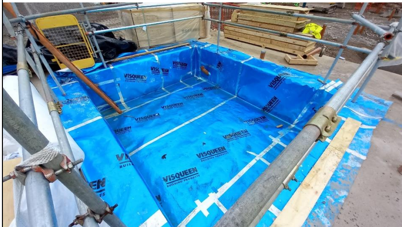
Photograph of the elevator shaft area lined and sealed with the Visqueen membrane. A service penetration at the top of the image is still requiring sealing.
