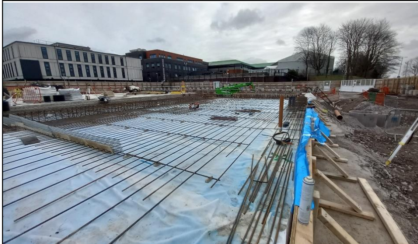
Photograph of the completed membrane installation, awaiting the concrete pour in the upper raft area. Photograph taken facing the east.
