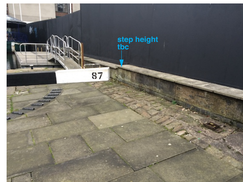
5**. Existing wall condition & step in coping height
