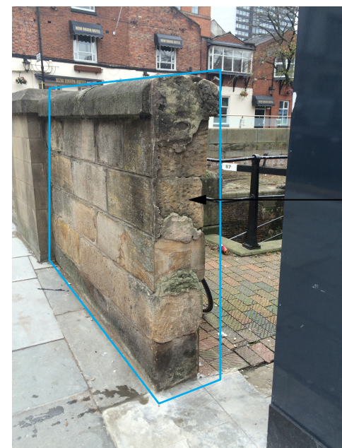
1. Wall outside site boundary to Princess Street bridge
