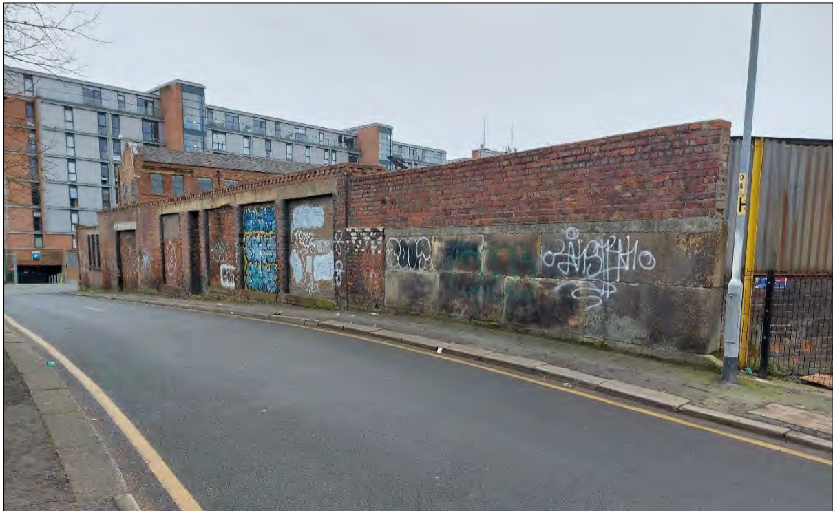
Plate 14 View of late 19 th -century wall of the former Phoenix Iron Works on Poland Street and the west wall of the former Poland Street canal bridge, looking south-west
