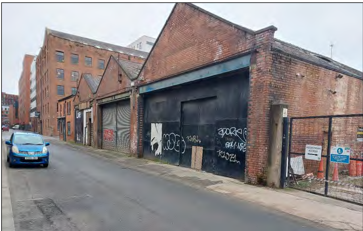
Plate 15 1920s garages fronting Jersey Street, looking west
