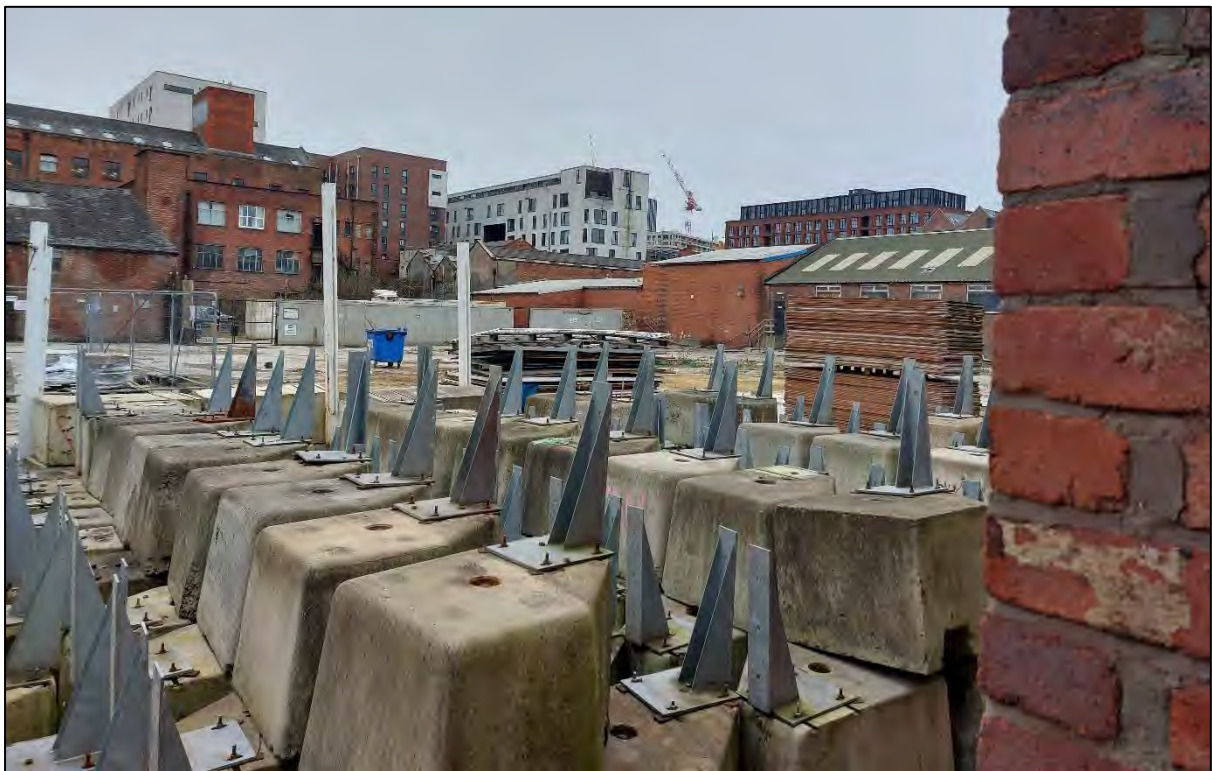
Plate 20 View of Site, looking north-west towards welfare cabins and 1920s garage
