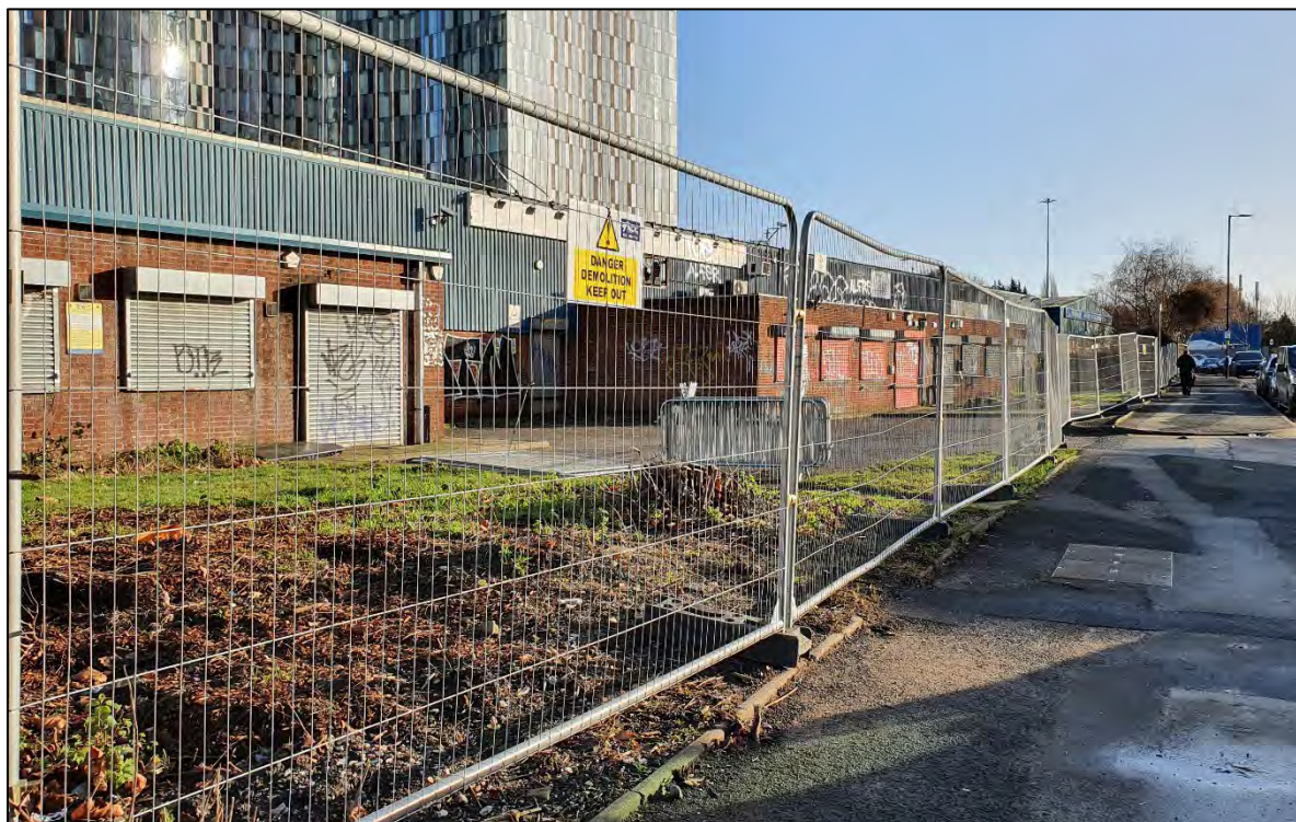
Plate 21 Showing the west elevation of the warehouse, with vegetation, flagstone pavements and hard-standing surfaces (looking south-east)
