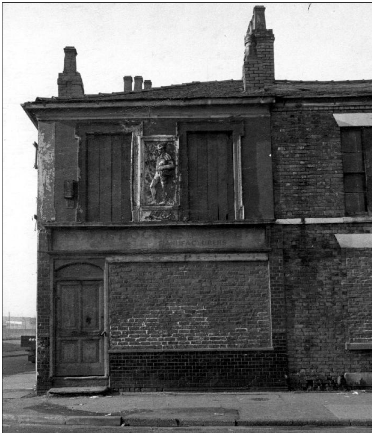
Plate 12 Photograph of No. 26 Great Jackson Street, situated at the junction of Melbourne Street, taken in the 1960s, courtesy of Manchester Local Image Collection
