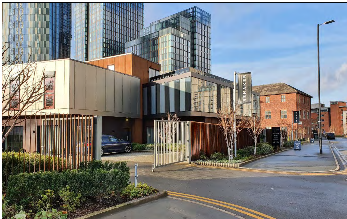
Plate 14 Showing the south-east and east elevations of the Renaker Marketing Suite and Gaddum House, with associated customer car parking (looking north-west)
