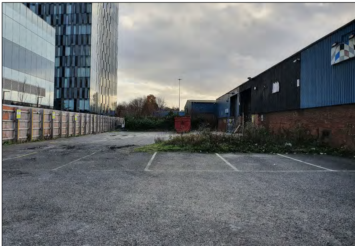
Plate 23 Showing the east elevation of the warehouse with wooden fencing to the east and former car parking area (looking south)
