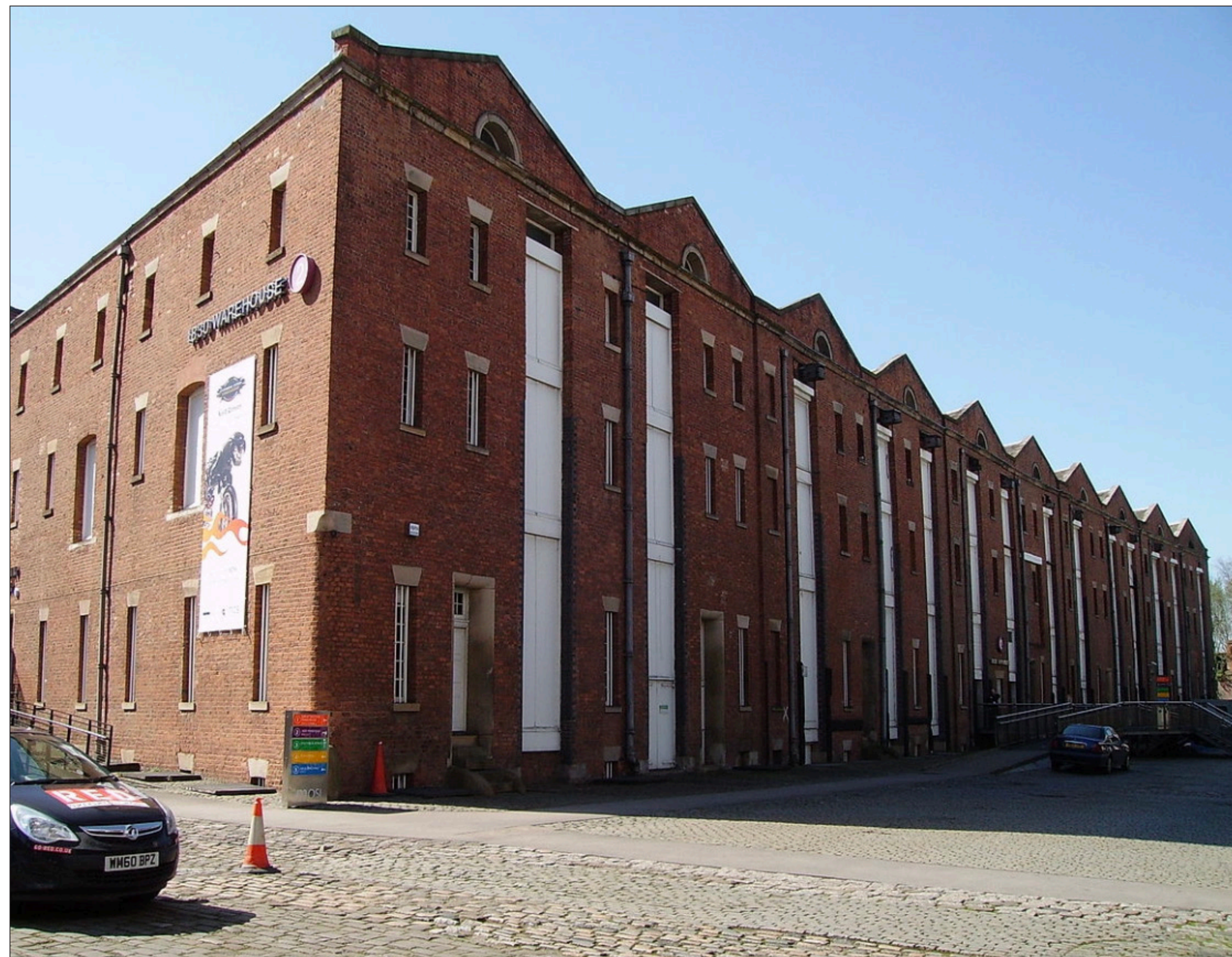
Image 4: Photograph of 1830s Warehouse from the yard side.
