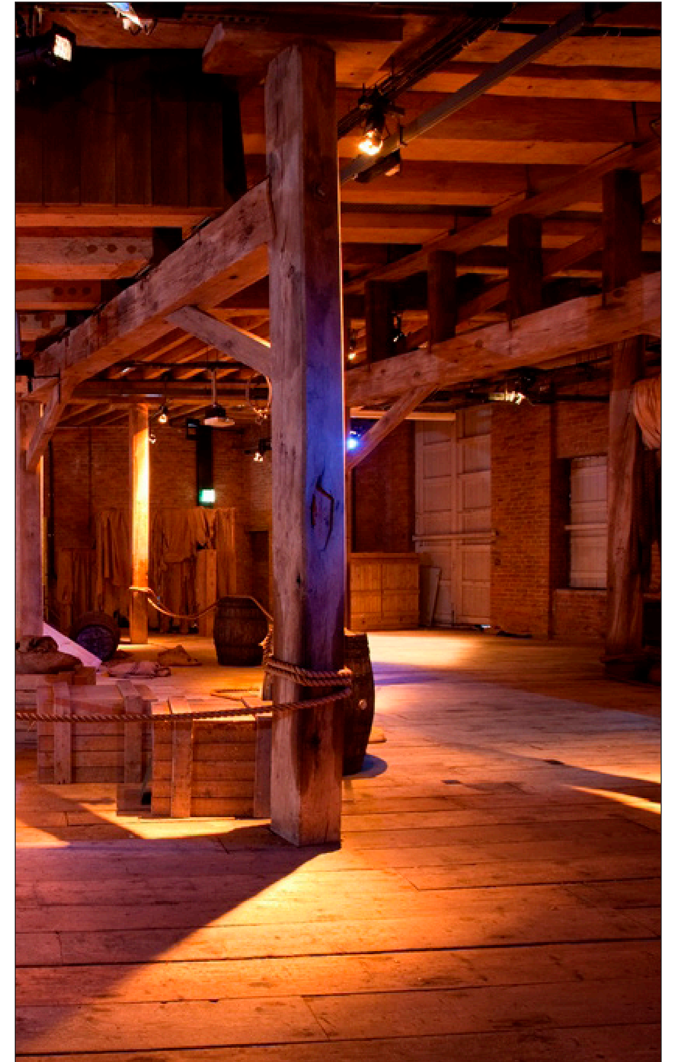
Image 6: Ground floor of 1830s Warehouse following conversion to museum.
