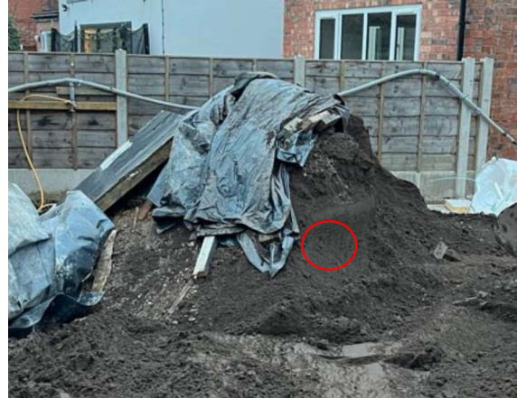
Photo 2: Topsoil Stockpile TP02
