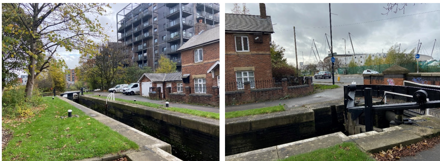
Figure 5.9: Setting of the Lock (Source: Authors Own, December 2022)
