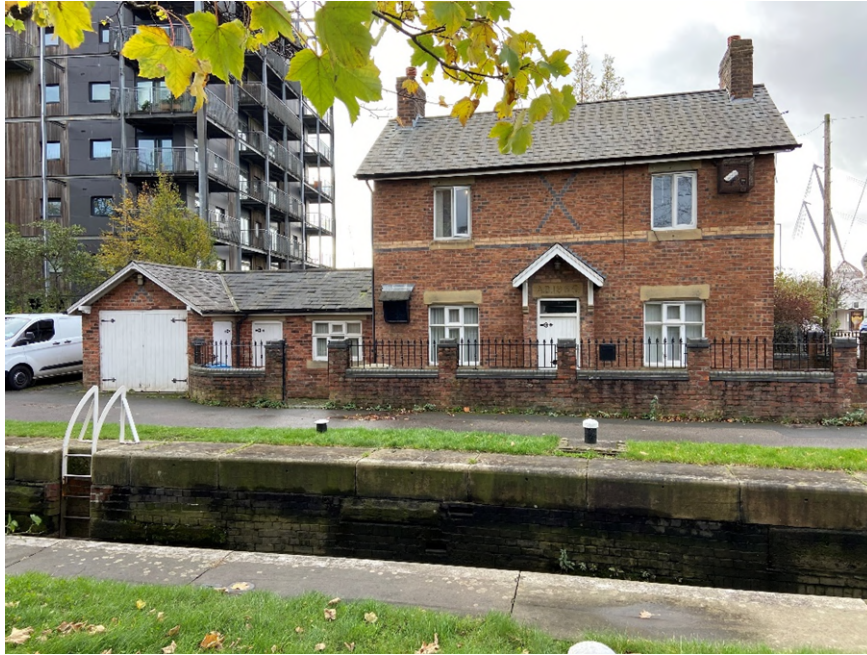
Figure 5.11: Principal Facade of the Lock Keepers Cottage (Source: Author's Own, 2019)
