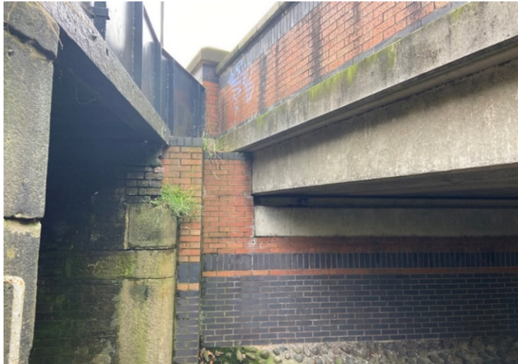
Figure 4.8: Mill Street Bridge (Source: Author's Own, November 2022)
