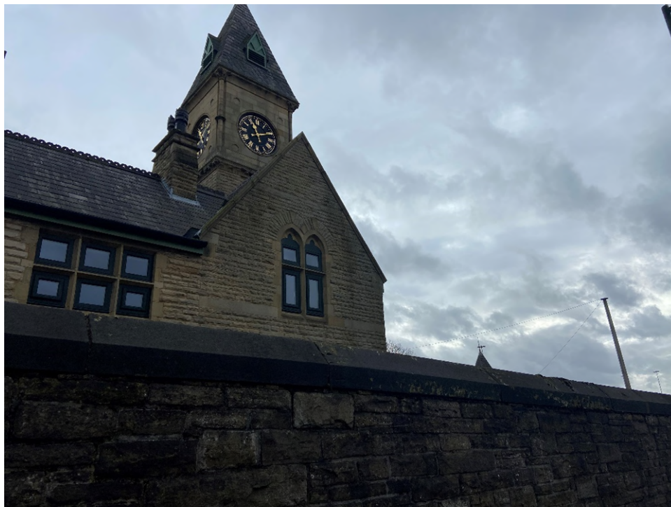
Figure 4.5: Cemetery Office at Phillips Park Cemetery Looking Towards the Site (Source: Author's Own, November 2022)
