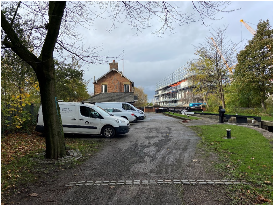
Figure 5.8: Ashton Canal Lock Number 7 with Roving Bridge Immediately East of Mill Street Bridge (Source, Author's Own, December 2022)
