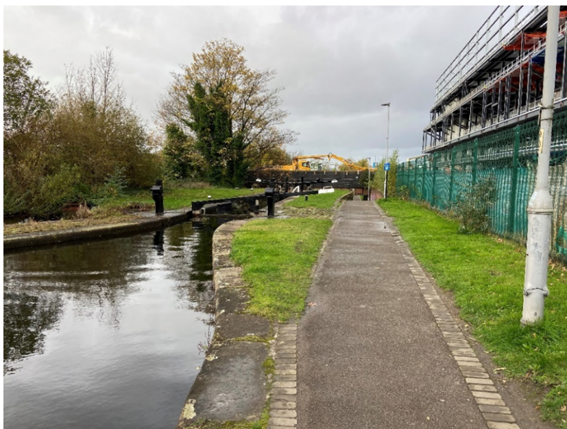
Figure 5.6: Ashton Canal Lock Number 6 Immediately East of Forge Lane Looking West (Source: Author's Own, December 2022)
