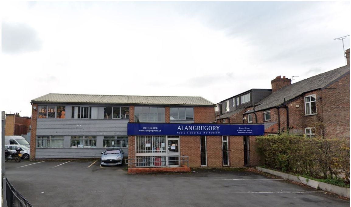
(Figure 5 – Close up photograph showing the front of the existing building)
