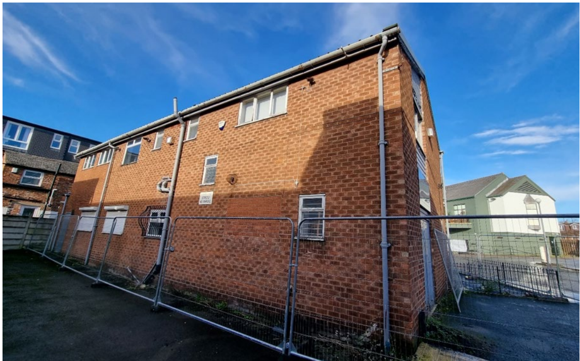
Figure 8 – Close up photograph showing the rear of the existing building)
