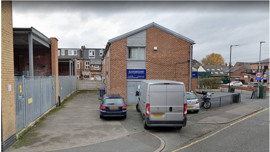
Figure 7 – Close up photograph showing the side of the existing building)
