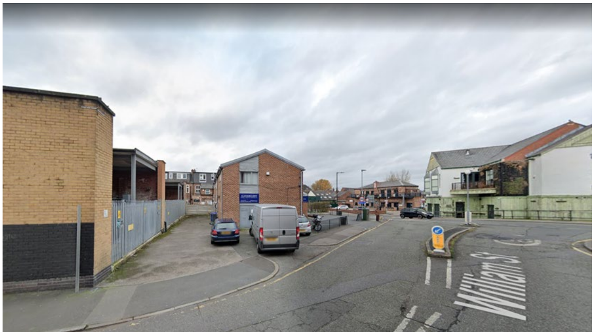
(Figure 6 – Photograph showing the side of the building and the wider street scene)
