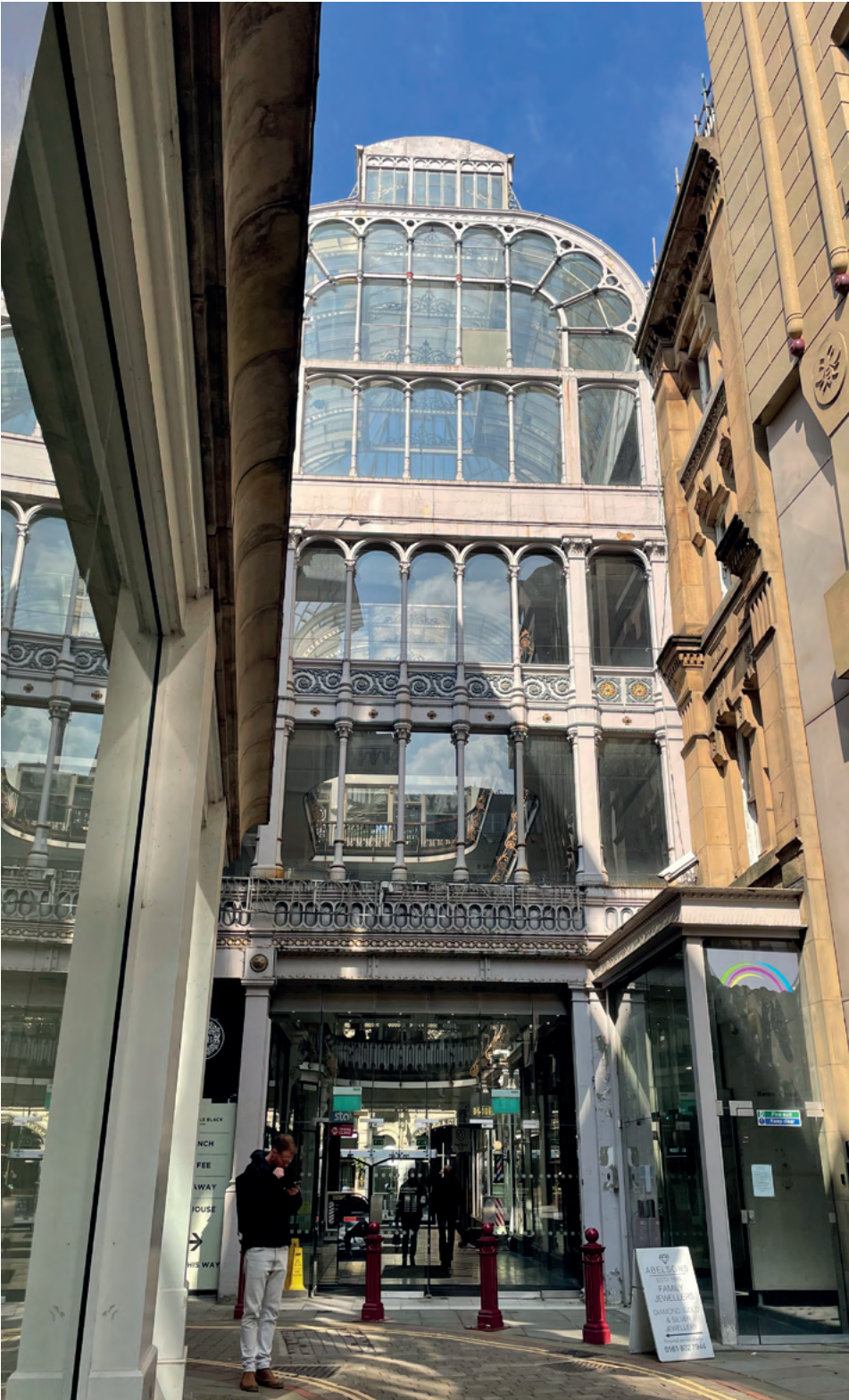
1 View looking to the principle, east, elevation
