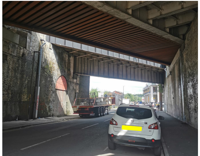
Figure 8: Dantzic Street under Rail Bridge
