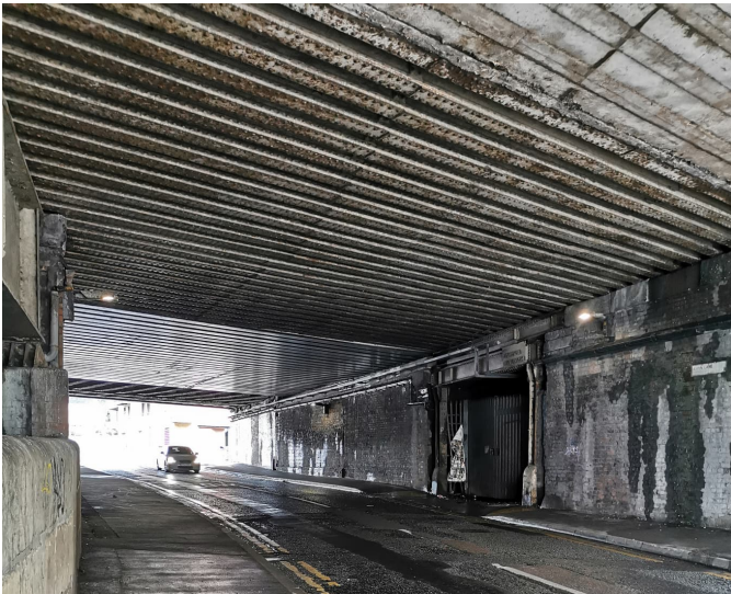
Figure 7: Red Bank under Rail Bridge
