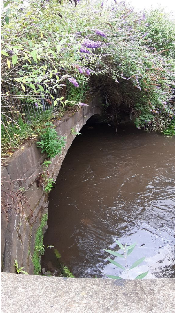
Figure 6-1 - Grade II listed Union Bridge, facing north west
