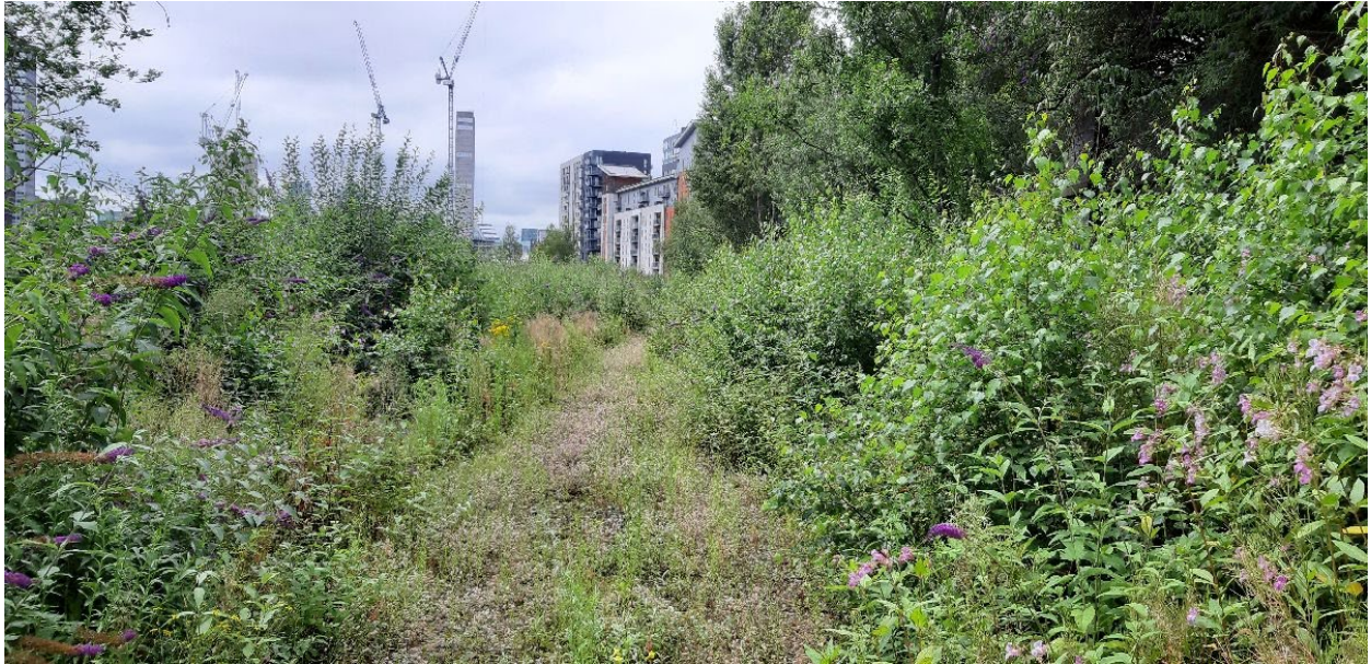
Figure 6-2 - View from the top of Red Bank Viaduct (WSP001) facing south west
