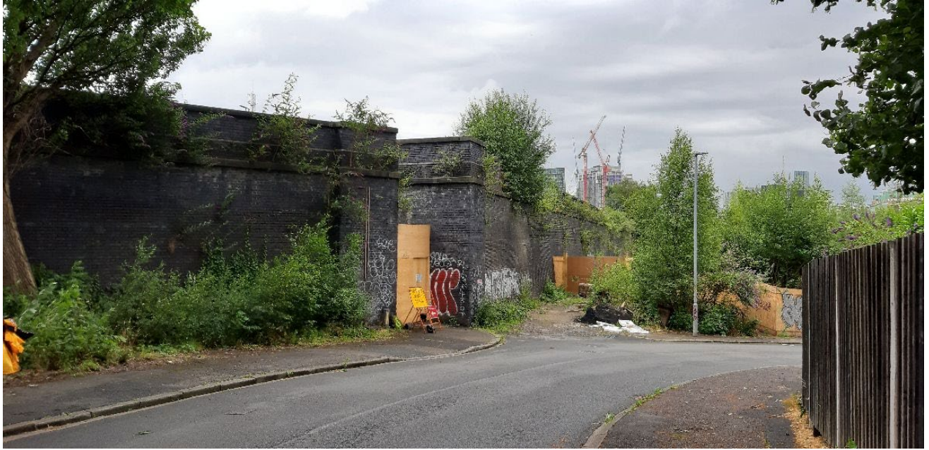
Figure 6-3 - View of south-west face of the Lancashire and Yorkshire Railway Viaduct
