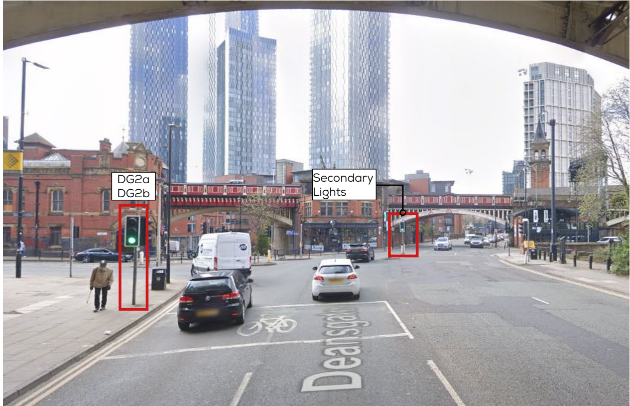
Fig. 36: Traffic Light Location
