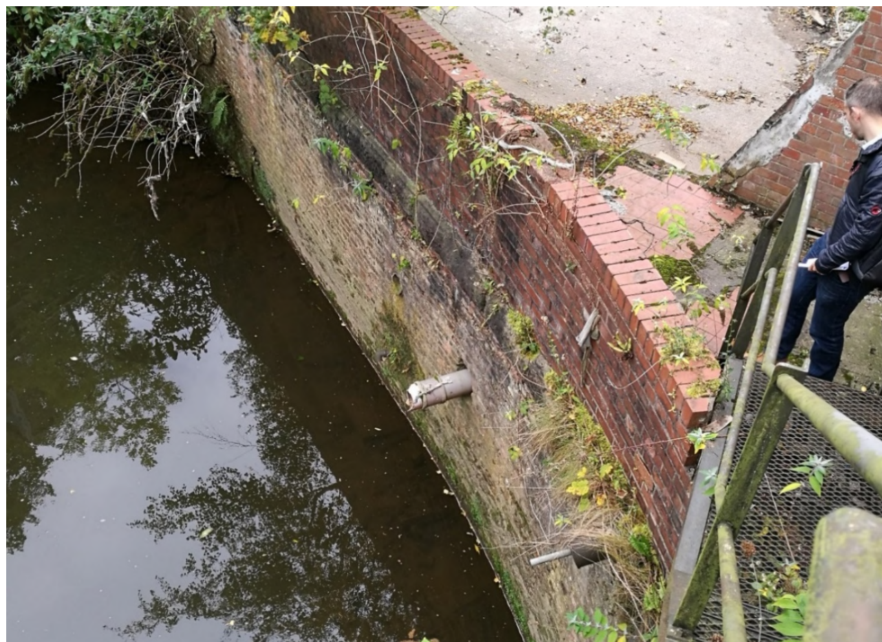
Figure 5-1 Existing Outfall Observed During Site Visit
