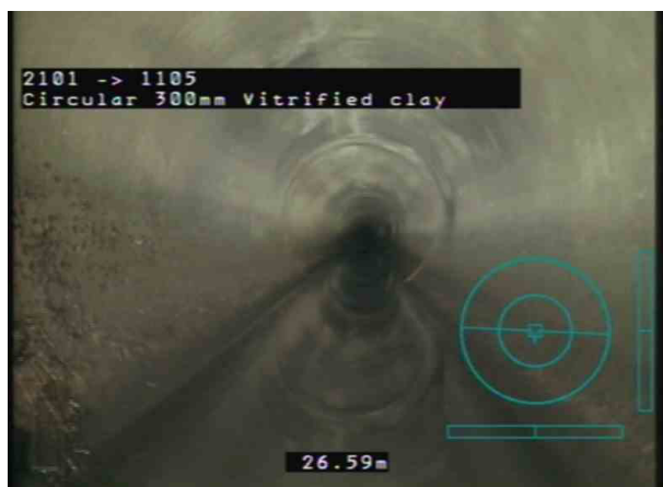
2101X_69d52bde-462e-4bab-beca-9a86779e0b75_20200109_082856_179.jpg, 00:11:34, 26.59 m Roots, fine
