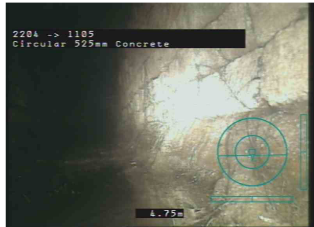
2204X_f012e500-f0fc-481b-b5e8-7461bc6394bf_20191218_220904_498.jpg, 00:07:33, 4.75 m Roots, tap
