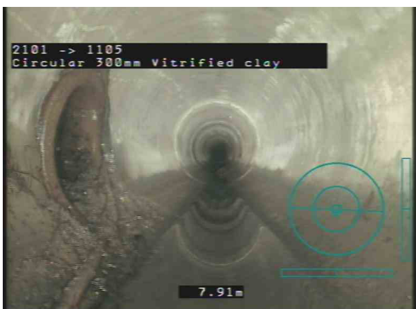
2101X_ba195ac0-e5d4-4fbc-bb1f-bffe23014324_20191218_23431_754.jpg, 00:04:33, 7.91 m Roots, tap
