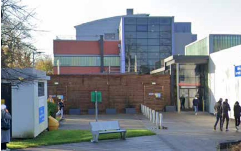
Existing Withington Hospital
