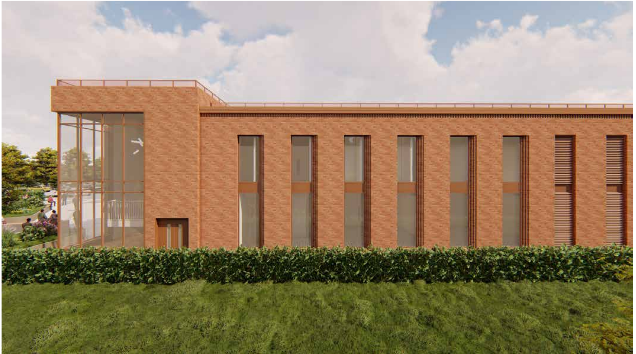
View of the elevation facing Fielden Road within the hospital site
