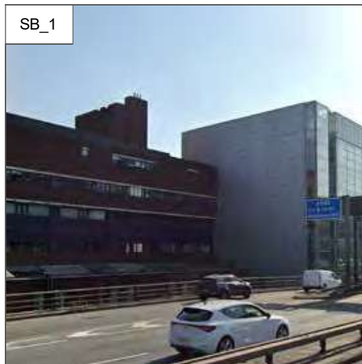
7. Existing Photograph Reference. View point from Mancunian Way Westbound
