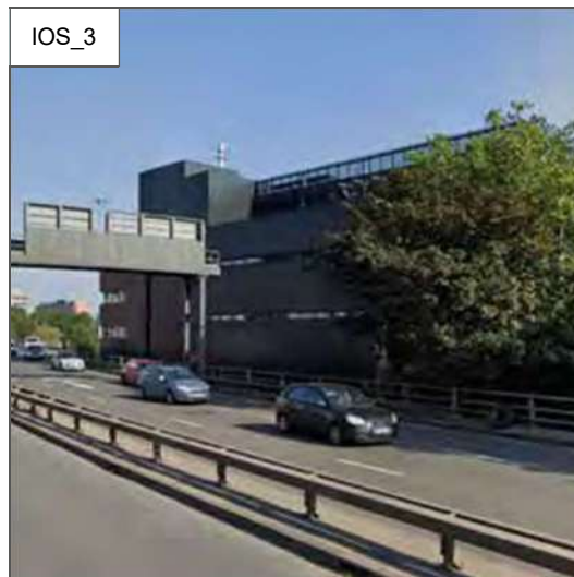
5. Existing Photograph Reference. View point from Mancunian Way Eastbound
