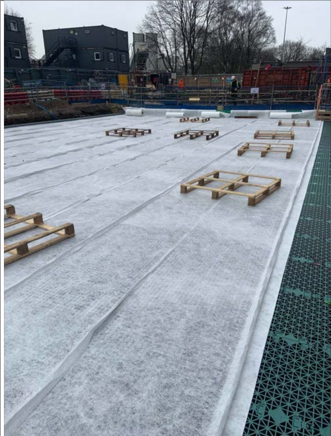
Photo 7 – Blue Roof Attenuation Crate Installation 28.03.23 viewed from ground level looking south
