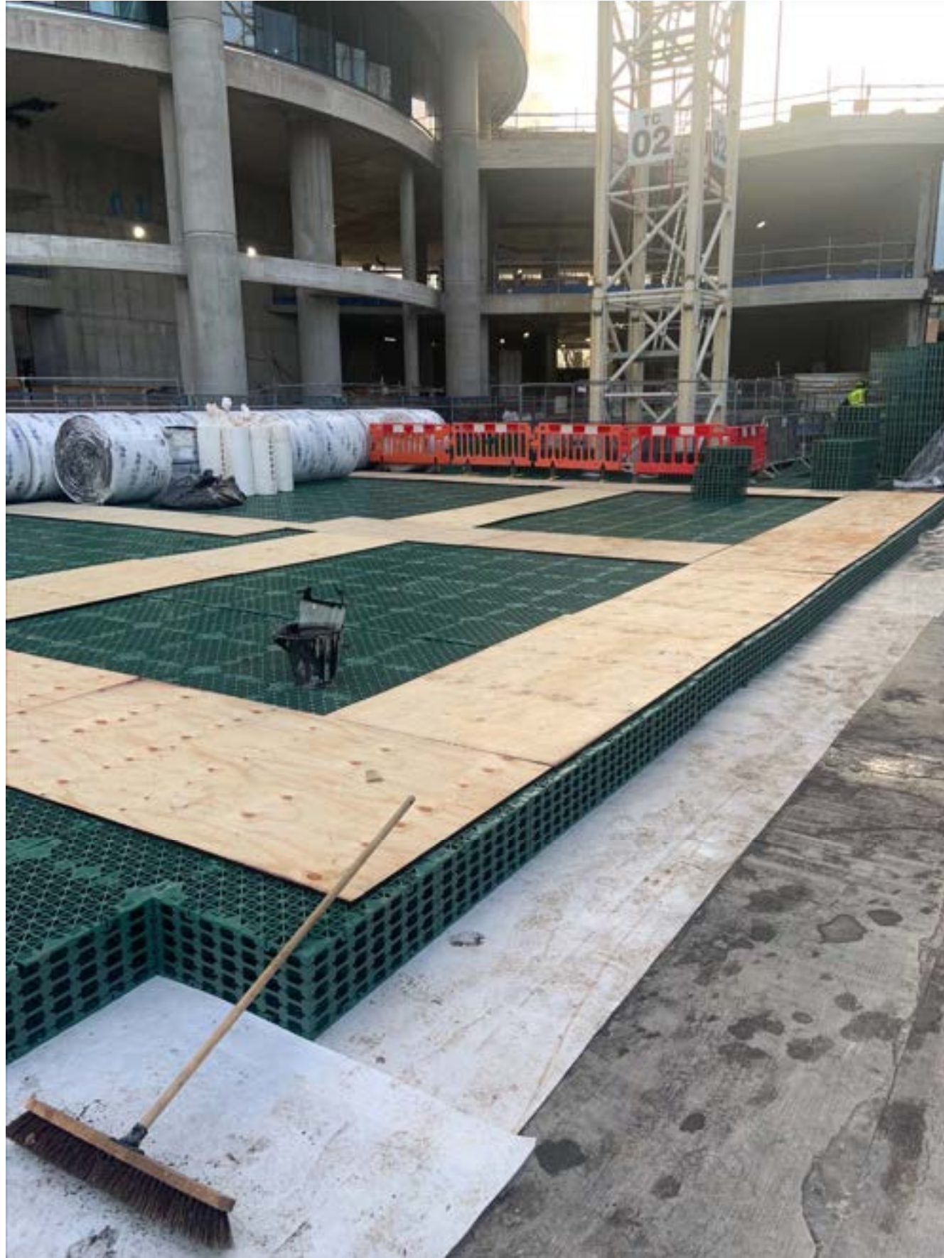
Photo 1 – Blue Roof Attenuation Crate Installation 23.01.23 viewed from ground level looking west
