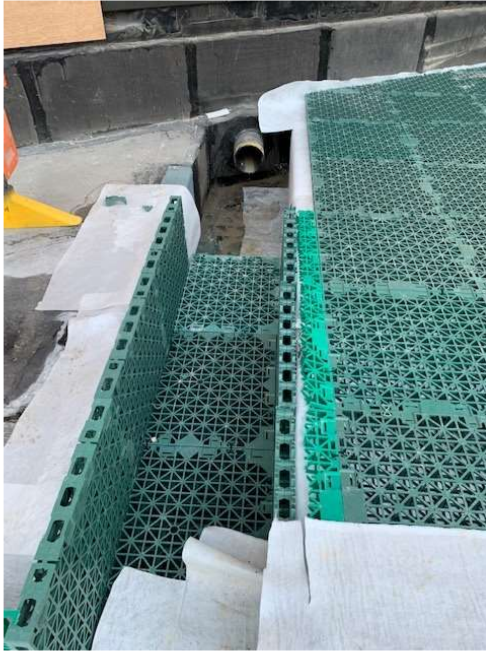
C5 Outfall 26/05/23 – Prior to installation of diffuser
