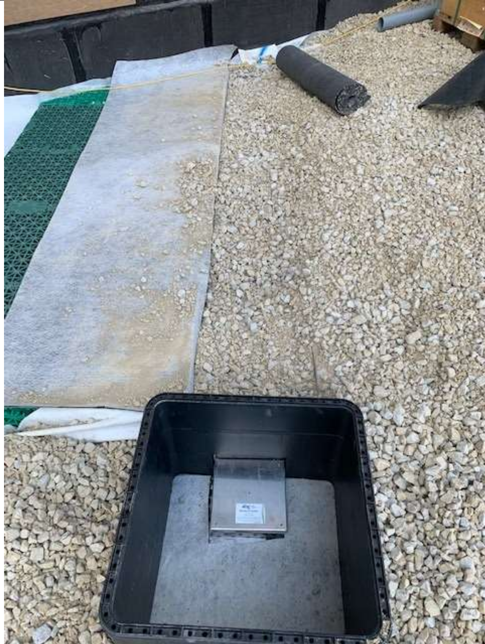
C5 Diffuser 05/06/23, after outfall pipework, diffuser, chamber and stone in place
