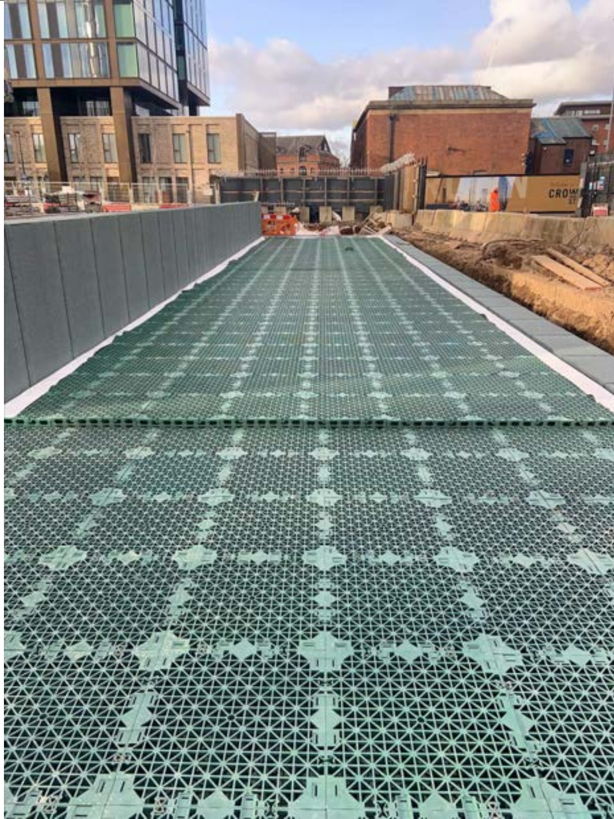
Photo 5 – Blue Roof Attenuation Crate Installation 09.02.23 viewed from ground level looking south
