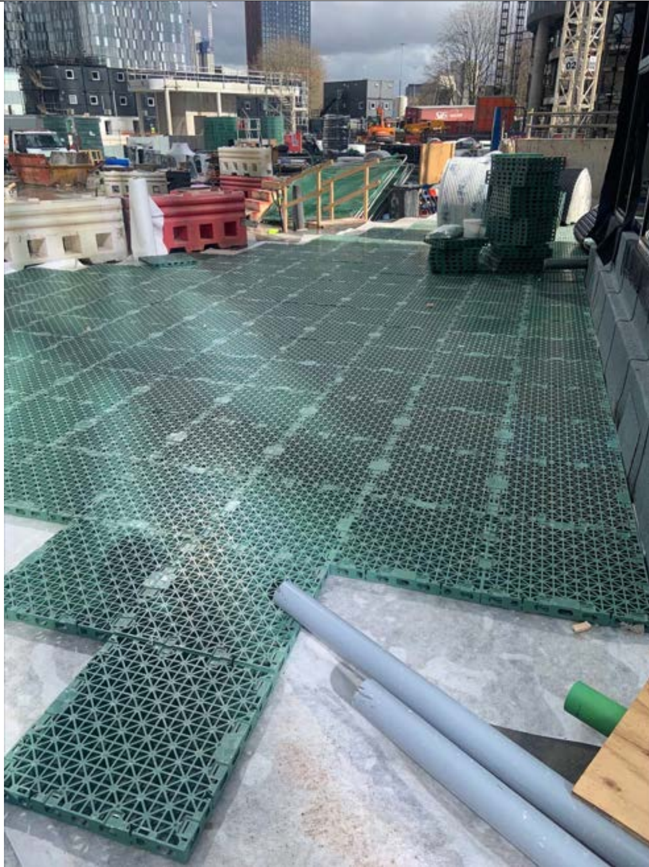
Photo 9 – Blue Roof 50mm Attenuation crate Installation around school 30.03.23 Viewed from School
