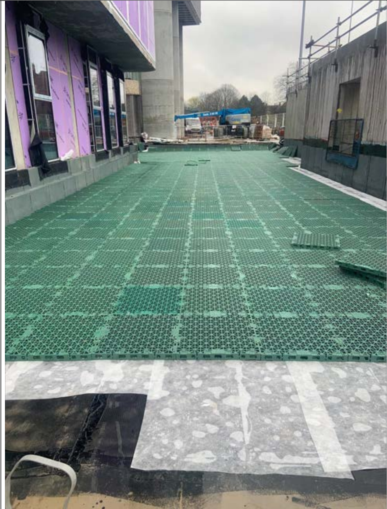
Photo 10 – Blue Roof 50mm Attenuation crate Installation around school 05.04.23 North of School
