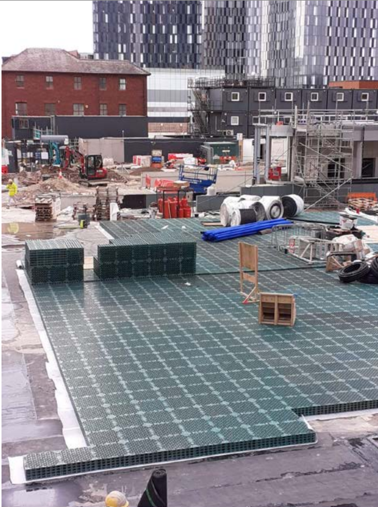
Photo 11 – Blue Roof Attenuation crate Installation 24.04.23 Viewed from School
