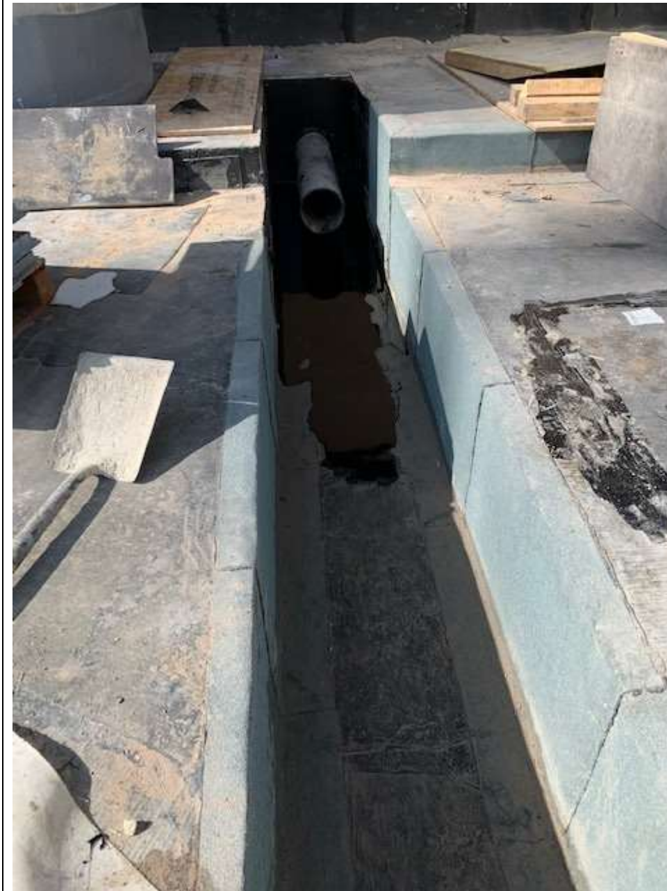
C4 Outfall 26/05/23 – Prior to installation of attenuation crate, drainage mat and diffuser
