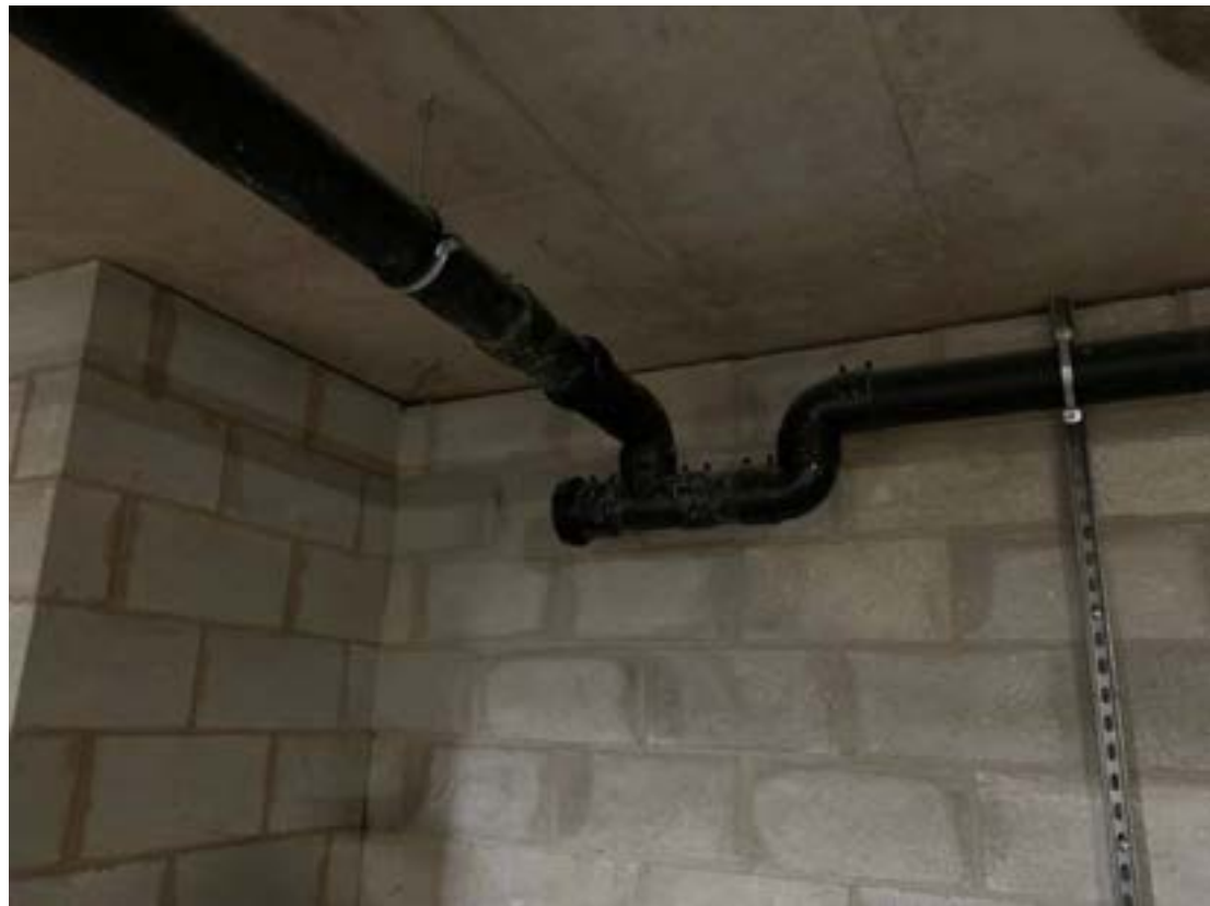
Photo 21 – B1 Level Underslung Drainage From Blue Roof Attenuation Crate To Main Drainage Spine
