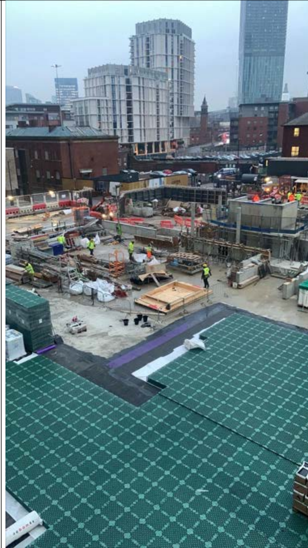
Photo 2 – Blue Roof Attenuation Crate Installation 24.01.23 viewed from C5 Level 2
