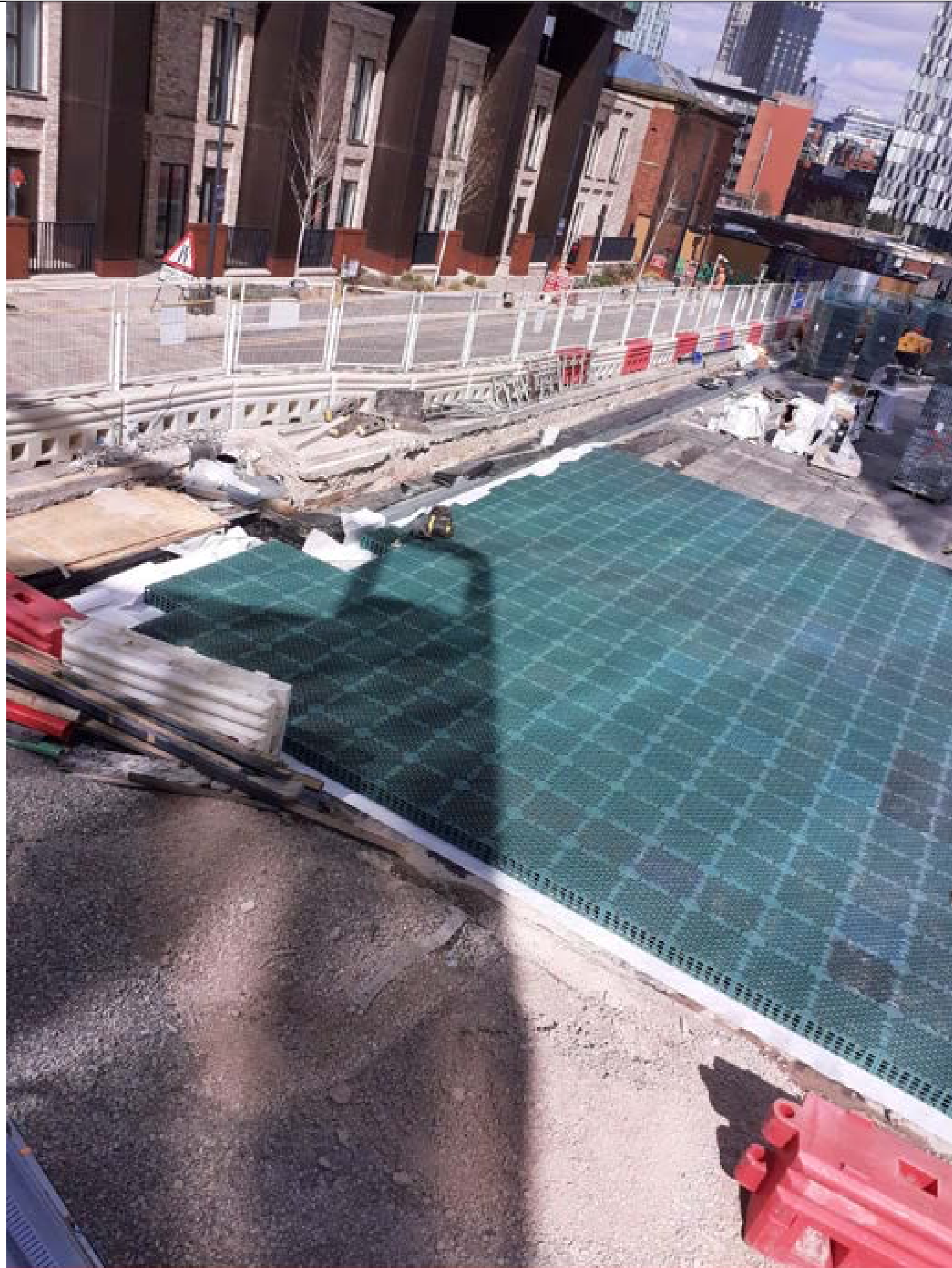
Photo 13 – Blue Roof Attenuation crate Installation 25.04.23 Viewed from School
