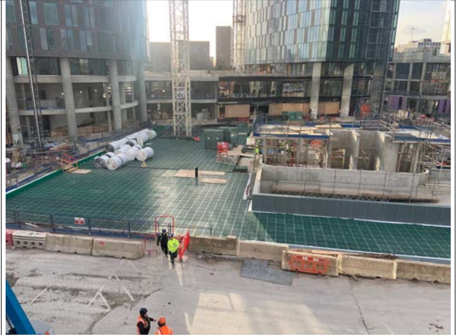
Photo 4 – Blue Roof Attenuation Crate Installation 09.02.23 viewed from Site Cabins looking West
