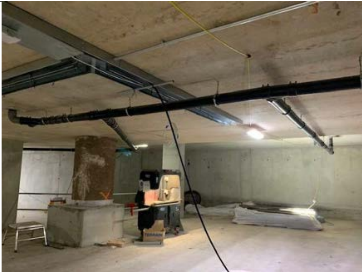
Photo 20 – B1 Level Underslung Drainage From Blue Roof Attenuation Crate To Main Drainage Spine
