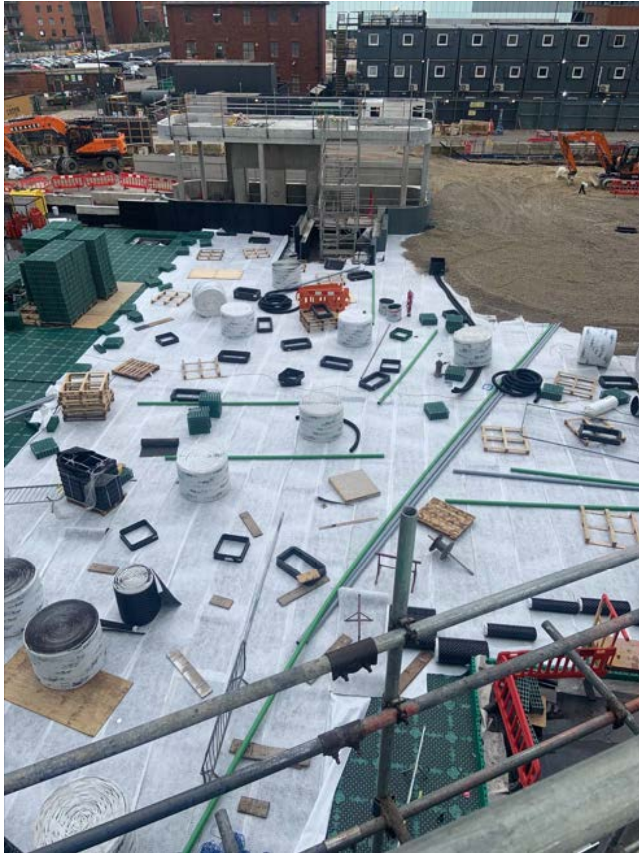
Photo 7 – Blue Roof ducting and stone Installation 29.03.23 Viewed from C4 Level 2
