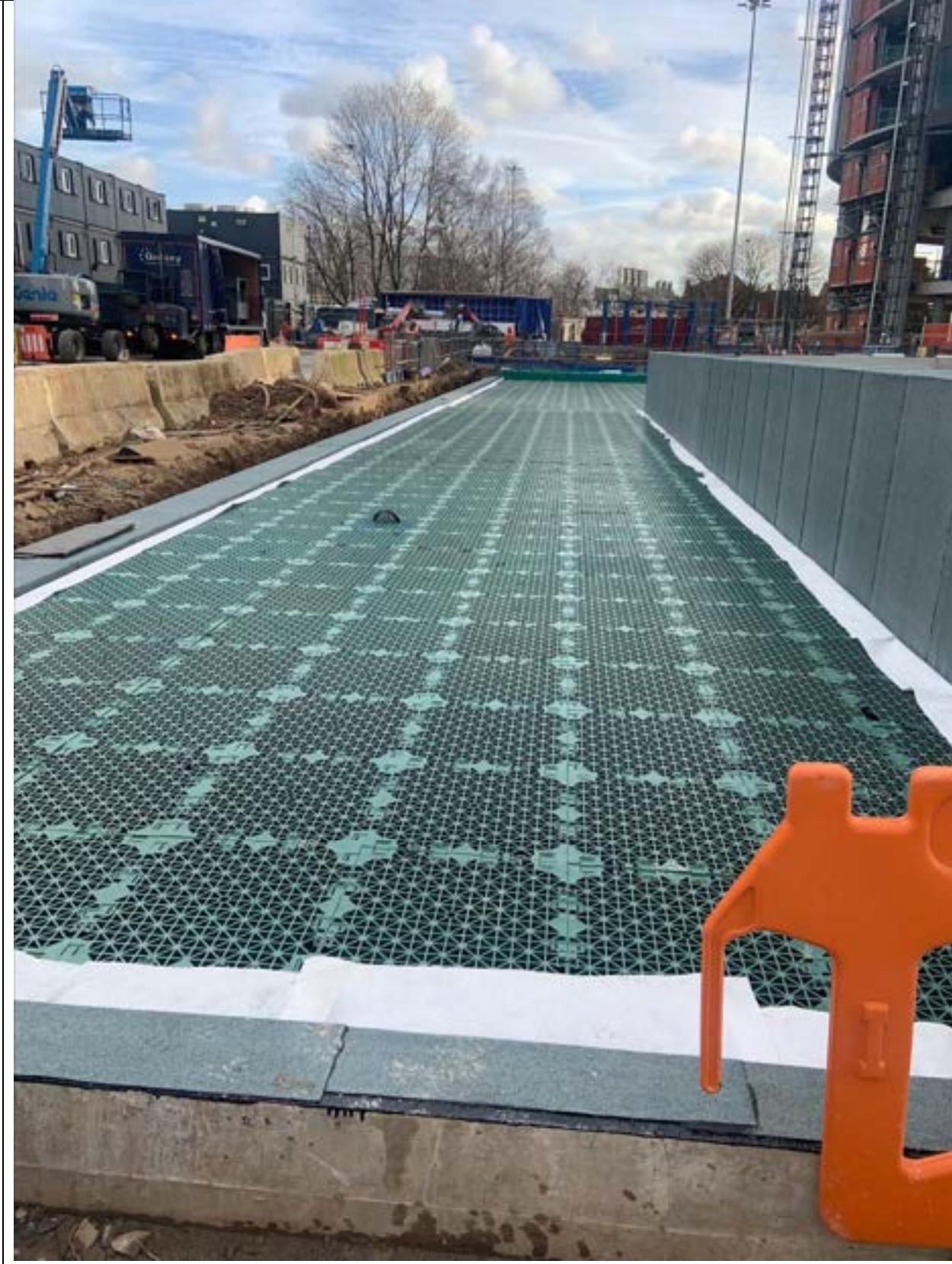
Photo 6 – Blue Roof Attenuation Crate Installation 09.02.23 viewed from ground level looking north
