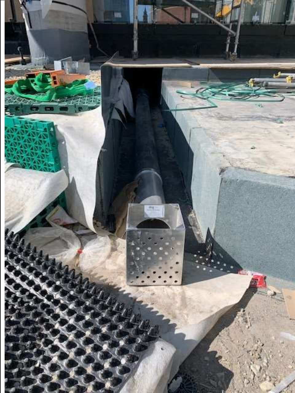
C4 Diffuser 05/06/23 after outfall pipework and diffuser in place
