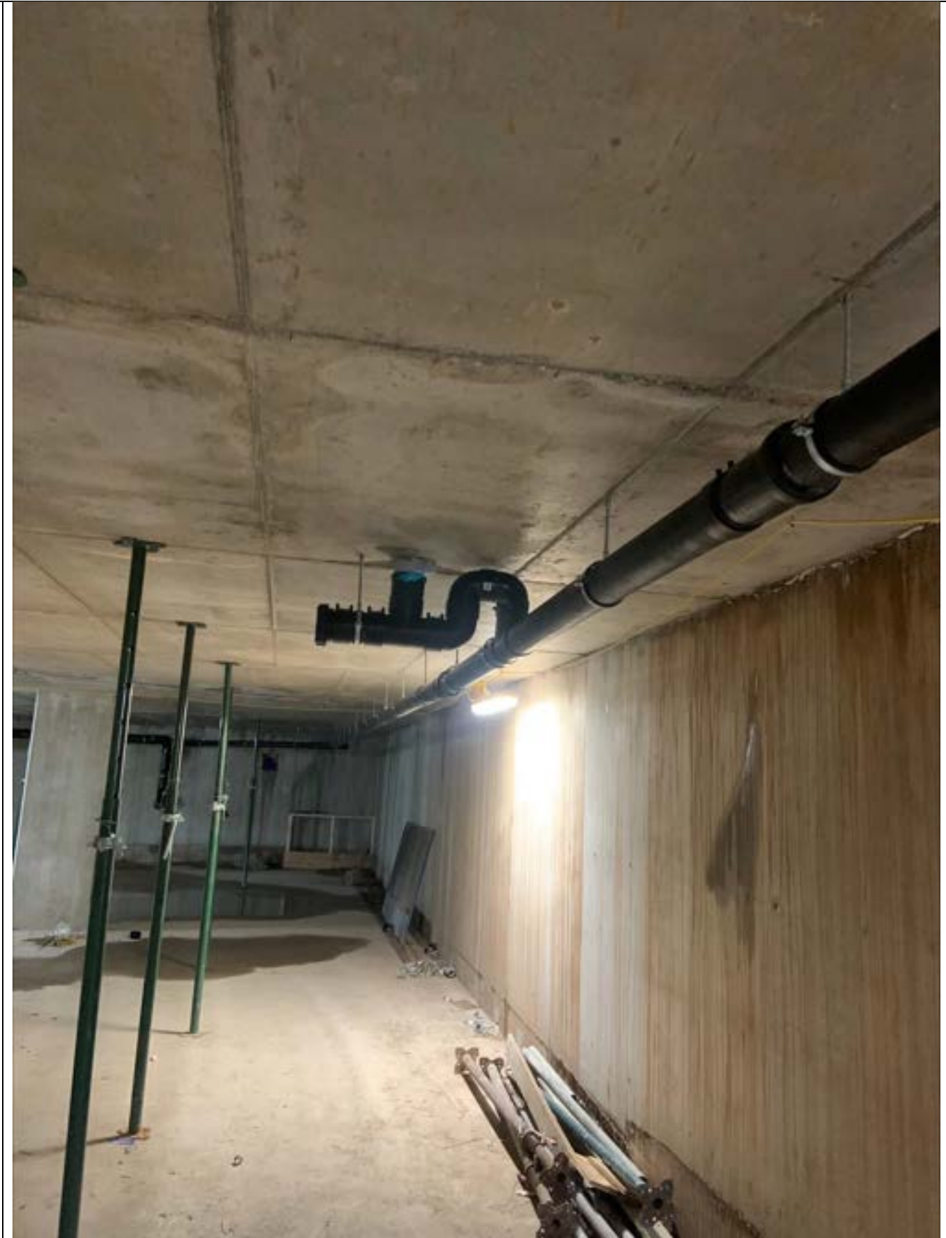
Photo 18 – Blue Roof Attenuation Crate Installation 09.02.23 viewed from Site Cabins looking West
