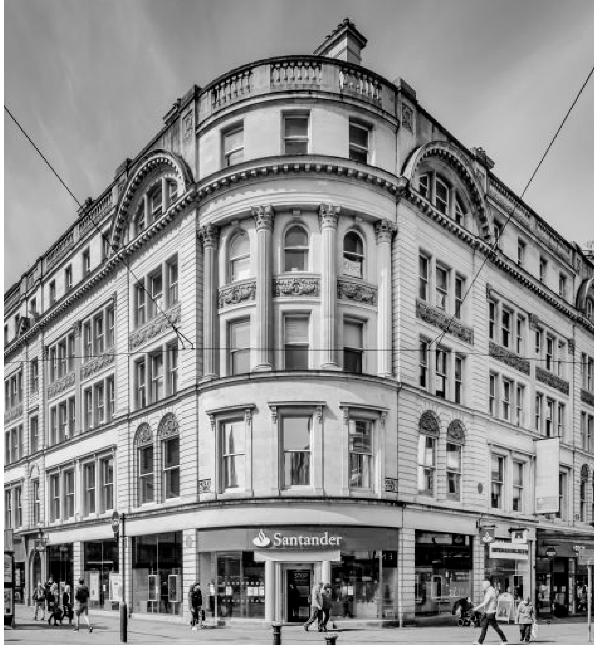
Figure 2 View of Royal Buildings from Market Street
