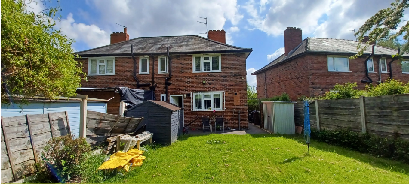
Figure 2. Rear view of property.
