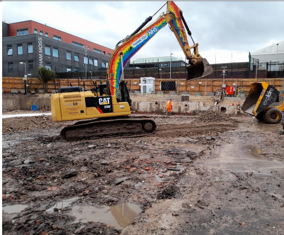
Photo 15: Excavation taken to the slab where VS17 was collected. LR01/LR02 was collected from the area underneath the slab (right of the photograph). Photograph taken facing the east on 20/10/2021.
