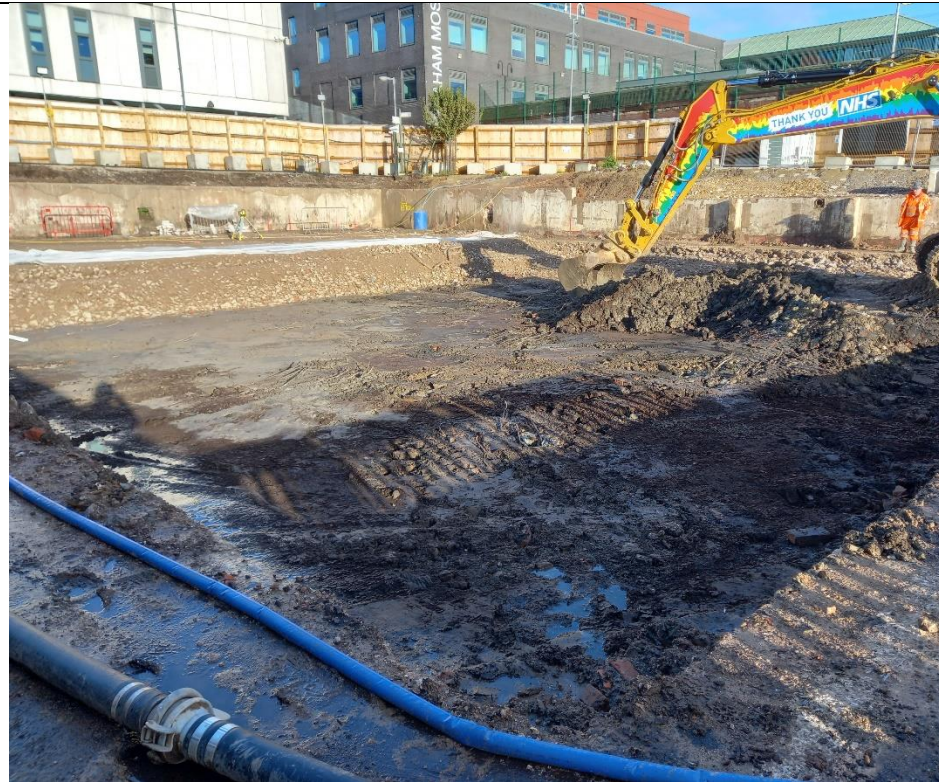
Photo 17: Excavation in the centre of the basement area (Zone D). Photograph taken facing the north-east on 20/10/2021.
