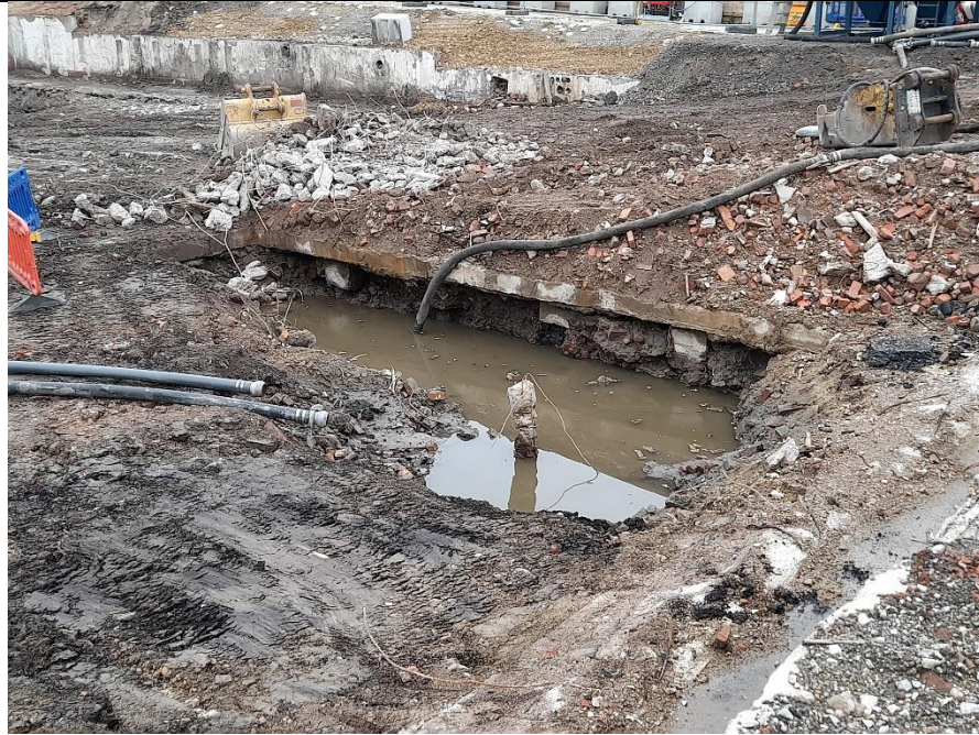
Photo 3: View of the groundwater within the Basement Area (the area where unexpected contamination was previous encountered. The water was pumped out of the pit and treated before discharge. Photograph taken facing the east / north-east on 18/10/2021.
