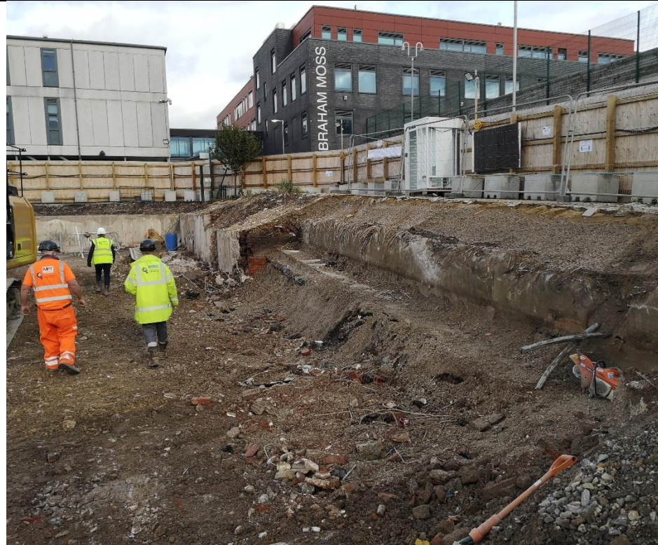
Photo 23: View of the removed eastern basement walls within the basement area. Photograph taken facing the north-east on 26/10/2021.
