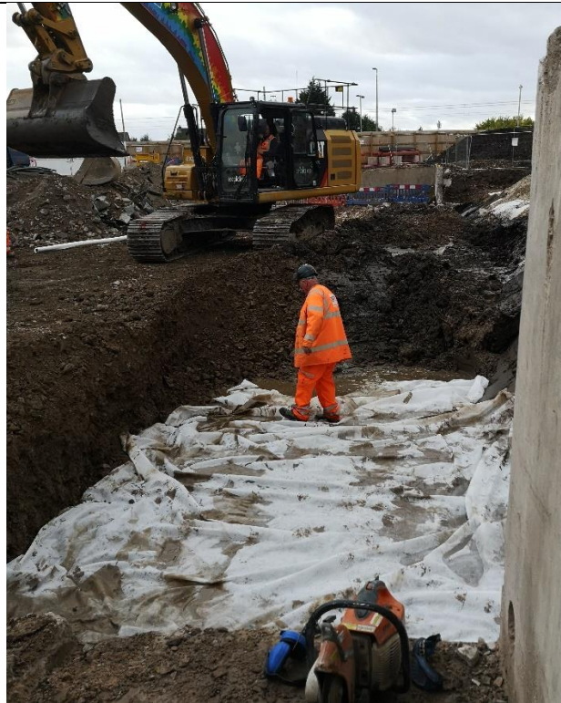
Photo 25: The new ramp excavation was lined with a geotextile on the 26/10/2021. Photograph taken facing the south.
