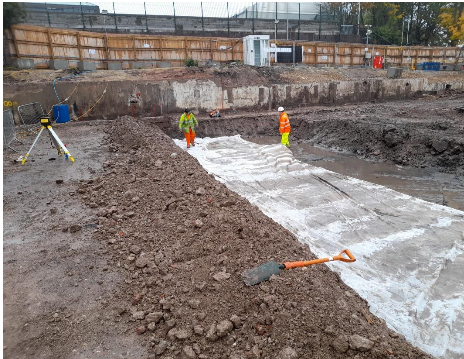
Photo 6: Contractor laying geotextile at the base of the excavation prior to backfilling with material. Photograph taken facing the east on 18/10/2021.
