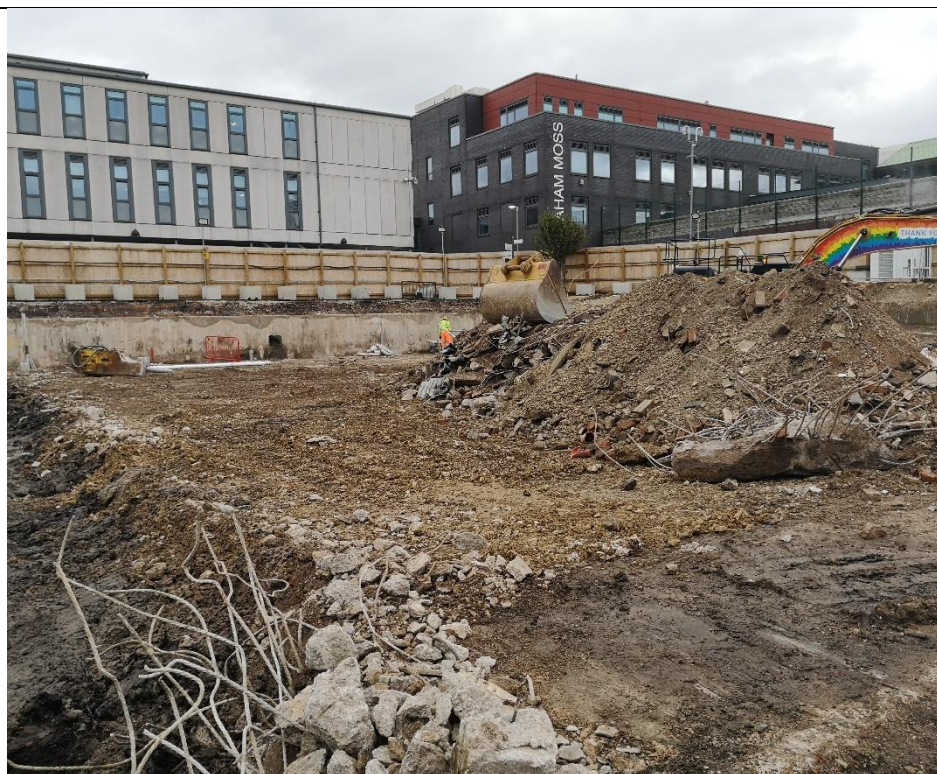
Photo 22: Temporarily stockpiled basement arising at the centre of the basement area. Photograph taken facing the north-east on 26/10/2021.
