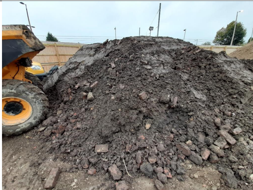
Photo 4: 'Hazardous' stockpile which was located to south-west of the Basement Area.
