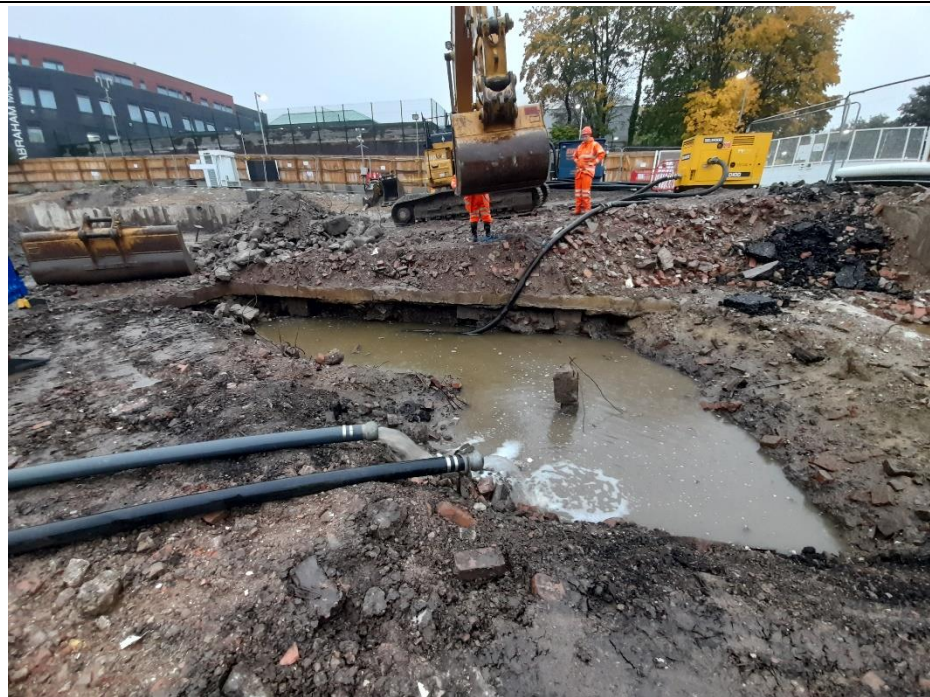
Photo 8: Groundwater / rainwater pumped out from an excavation north of the basement into the pit towards the south of the basement to be pumped out and treated via SiltBuster and pH regulating system prior to discharge. Photograph taken facing the east / south-east on 19/10/2021.
