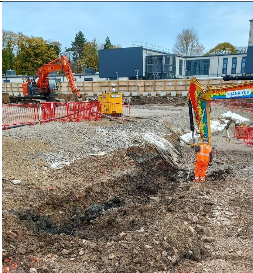
Photo 42: Ground conditions beneath the former concrete slab in the west / south-west of the basement. Photograph taken facing north on 09/11/2021.
