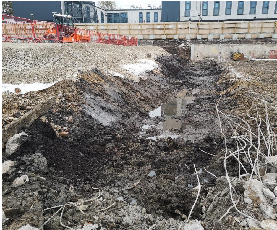
Photo 21: View of the ground conditions beneath the removed western basement wall. Photograph taken facing the north on 26/10/2021.
