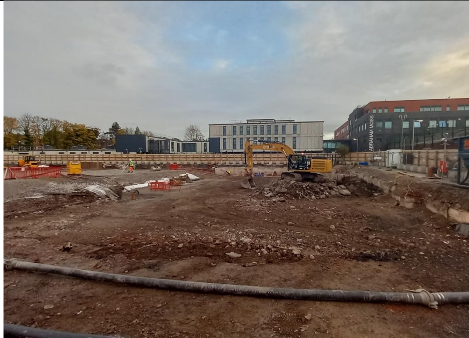
Photo 41: View of the basement area (beneath the concrete slab). Photograph taken facing the north and north-east on 09/11/2021.
