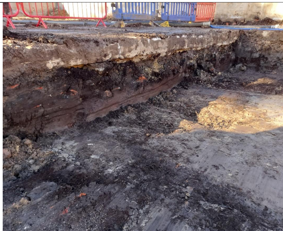
Photo 18: Zone D - Ground conditions approximately 1m north of the prior encountered contamination (August 2021). Ground prior to being lined and backfilled. Photograph taken facing the west on 21/10/2021.
