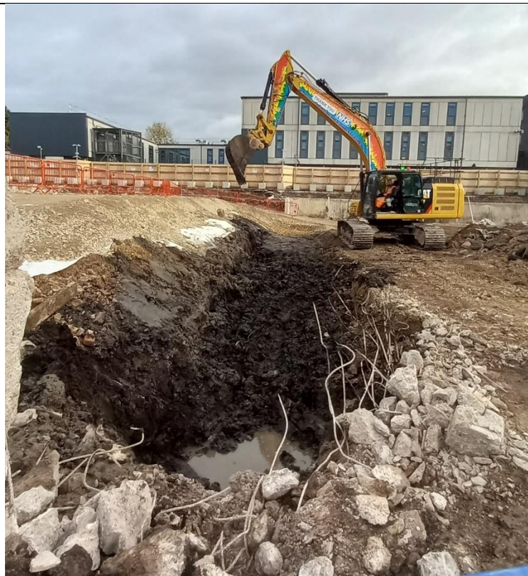
Photo 26: Ground conditions beneath and in proximity to the western basement wall following removal. Photograph taken facing the north / north-east on 27/10/2021.
