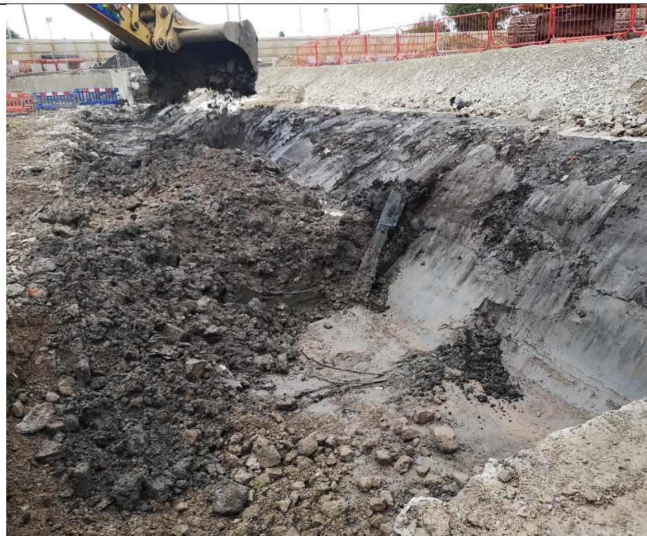
Photo 24: Excavation in the north-west of the basement area to allow for a new access ramp to the basement. Photograph taken facing the south / south-west on 26/10/2021.
