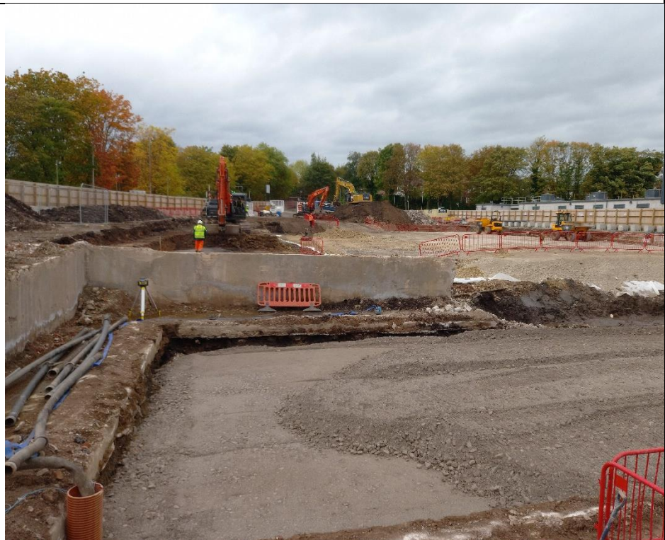
Photo 36: Backfill spread across Zone E in layers. Photograph taken facing the west on 28/10/2021.
