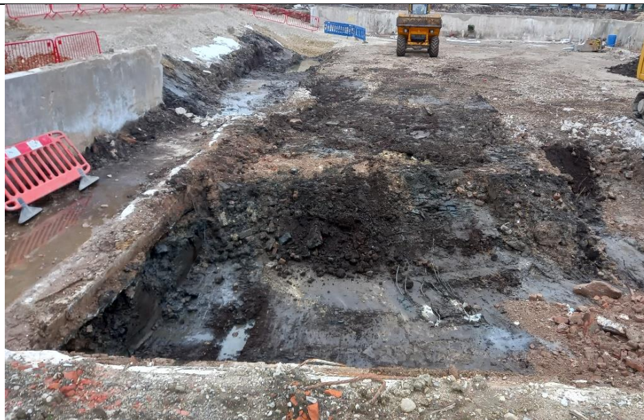
Photo 32: : View of excavated Zone E (in the south-west of the Basement Area). Photograph taken facing the north-east on 27/10/2021.
