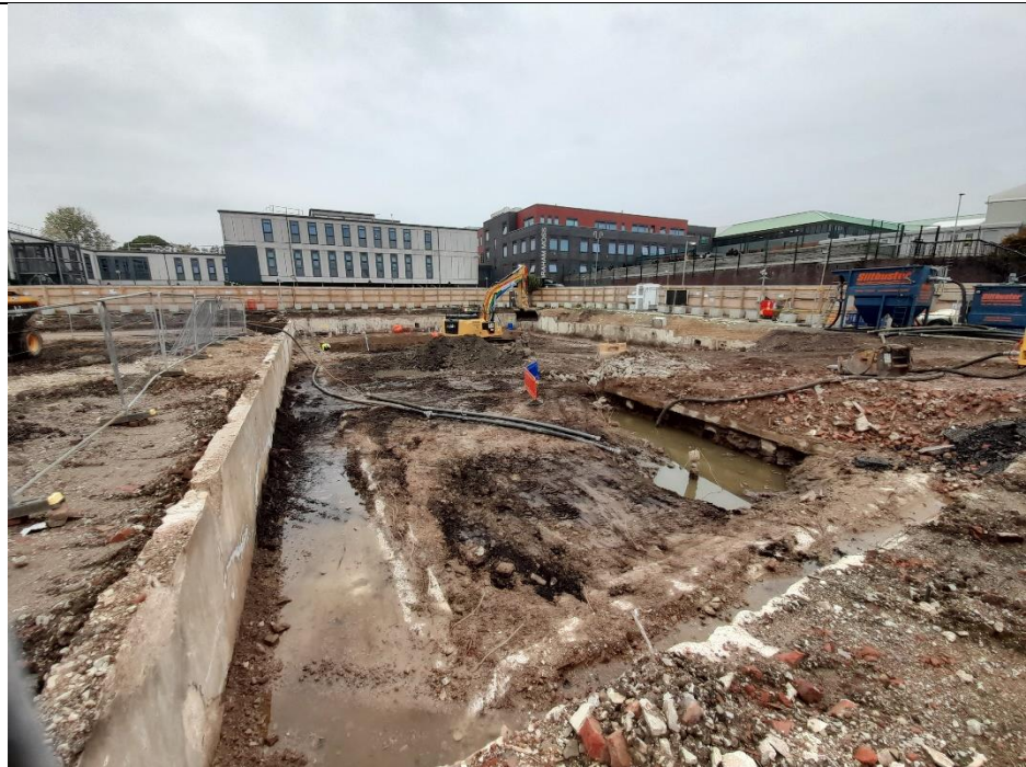
Photo 5: View of the Basement Area facing the north / north-east on the 18 th October 2021.
