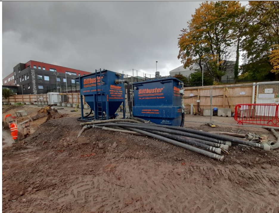
Photo 11: On-site water treatment system, located to south-east of the basement area. Photograph taken facing the north-east on 20/10/2021.
