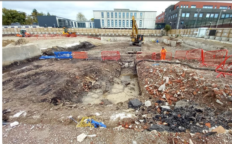
Photo 28: Water had been pumped out of the pit towards the south of the basement to allow for works within this area. Photograph taken facing the north / north-east on 27/10/2021.
