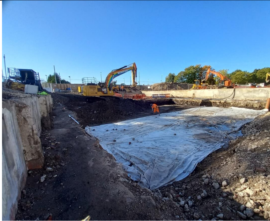
Photo 19: Centre of the basement area excavation lined with a geotextile. Photograph taken facing the south / south-west on 21/10/2021.
