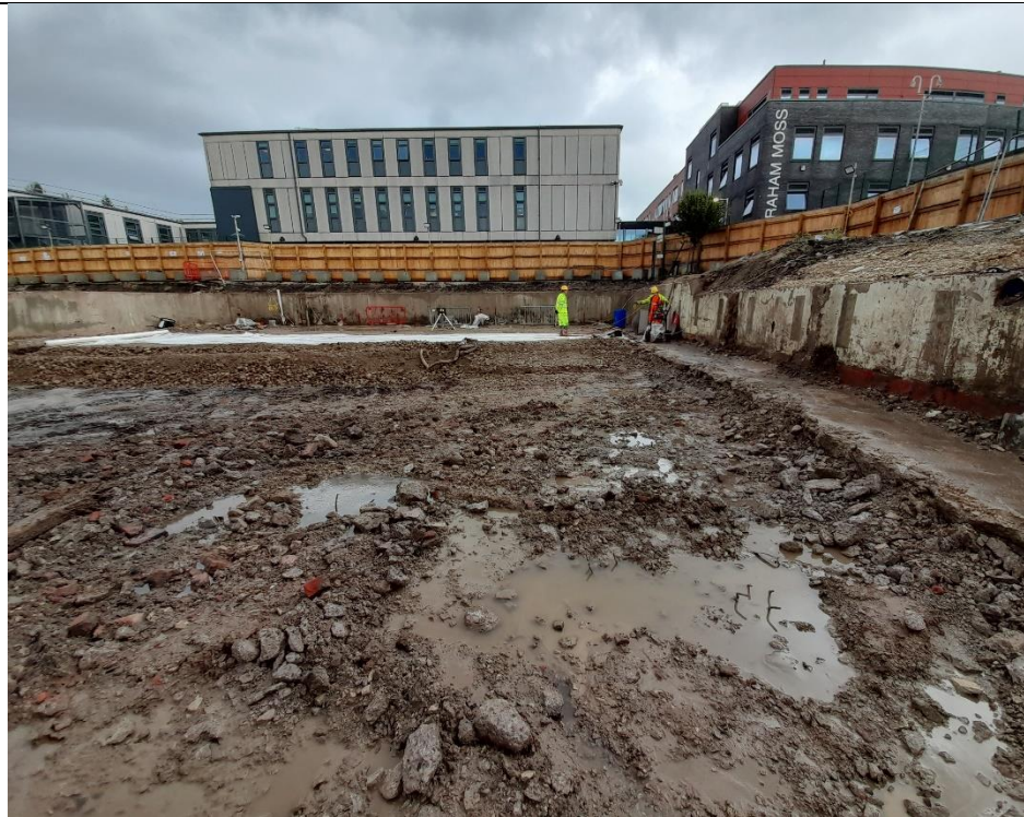
Photo 14: Excavation within the centre of the basement area with visible walls around the basement perimeter. Photograph taken facing the north / north-east on 20/10/2021.
