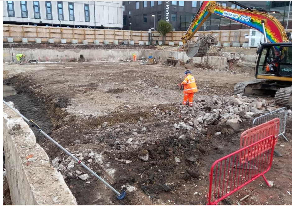
Photo 29: Breaking out of concrete strip towards the south-west of the basement. Photograph taken facing the north-east on 27/10/2021.
