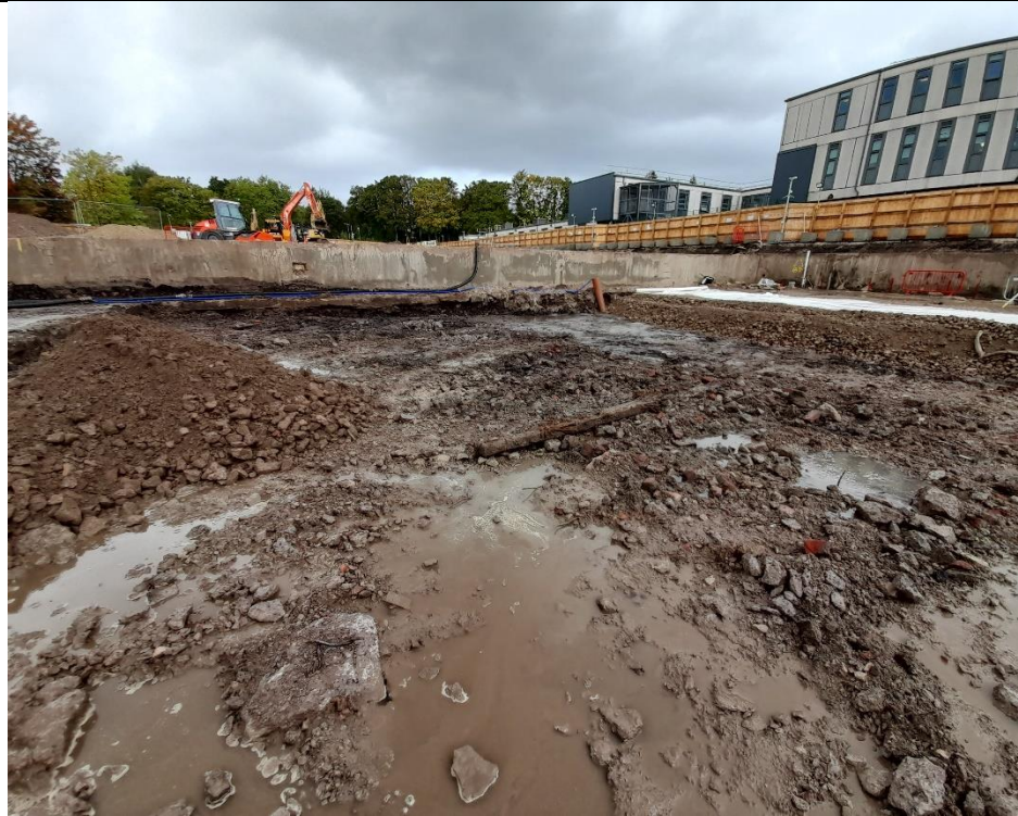
Photo 13: Excavated area in the centre of the basement area. Photograph taken facing the north-west on 20/10/2021.
