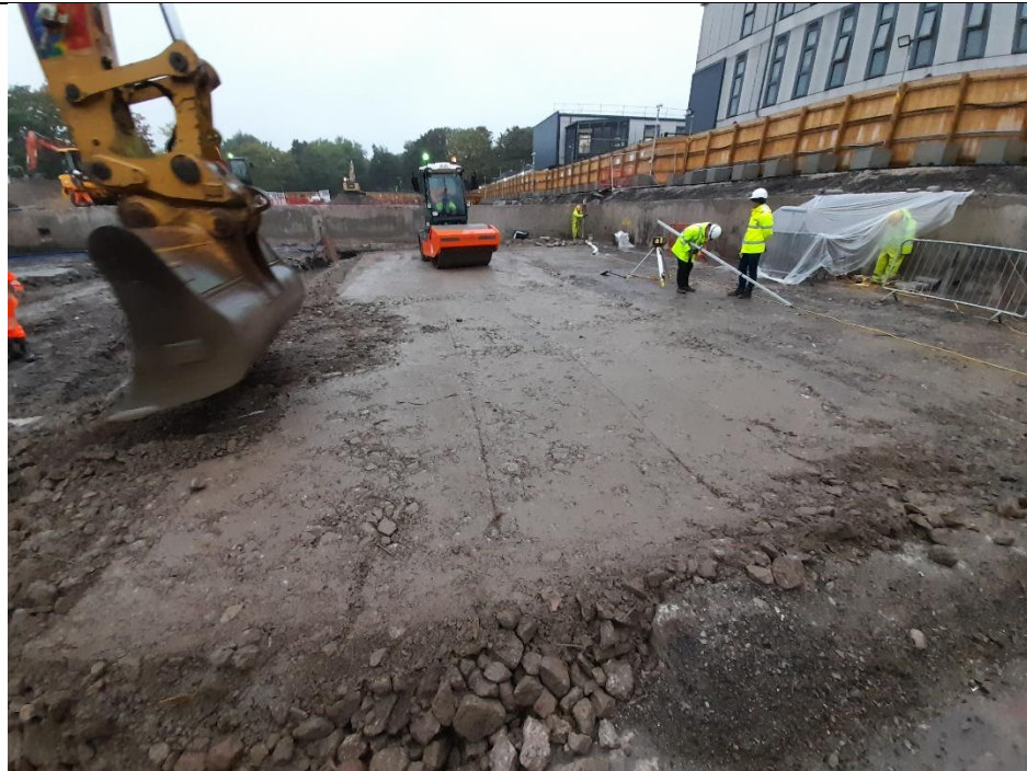
Photo 7: Roller compacting the backfill to form new foundation levels. Photograph taken facing the north-west on 19/10/2021.
