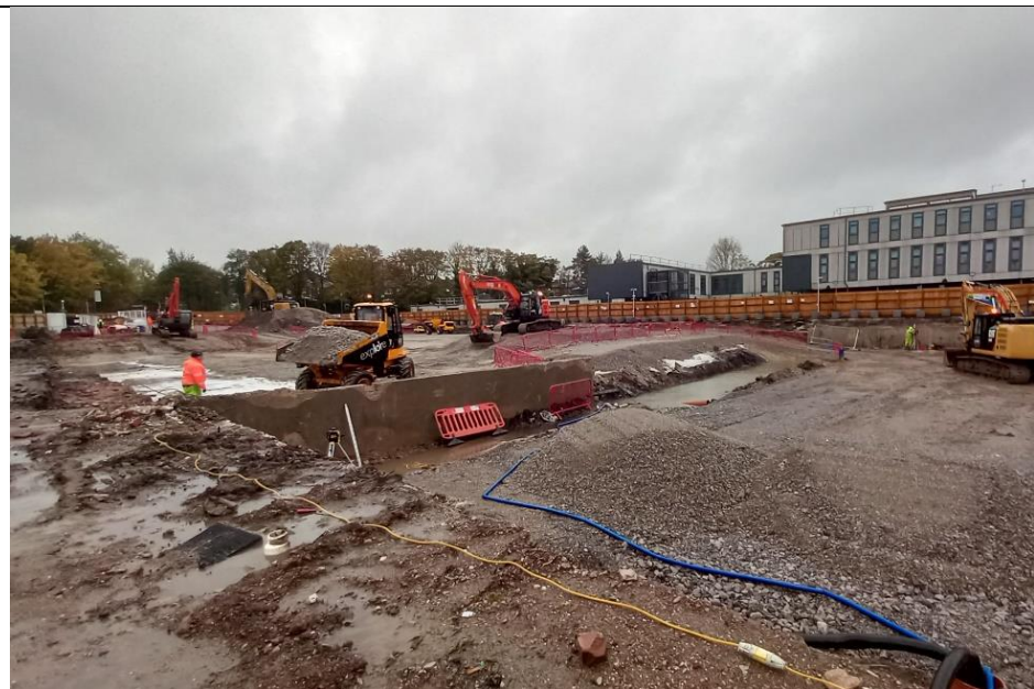
Photo 39: View of the basement area facing the north-east and east on 01/11/2021.
