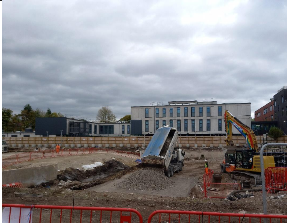
Photo 35: Imported aggregates used for backfill in the southern area of the basement. Photograph taken facing north / north-east on 28/10/2021.
