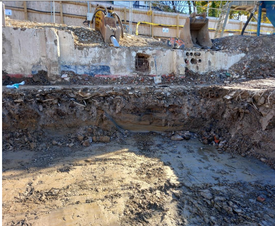
Photo 20: View of the ground conditions towards the east of the basement area. Photograph taken facing the east on 21/10/2021.
