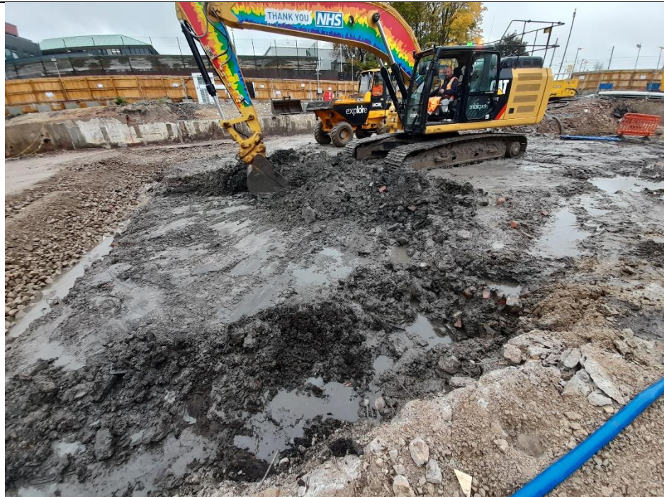
Photo 9: Ground conditions towards the north of the basement area following the pumping out of the groundwater. Photograph taken facing the south-east on 19/10/2021.
