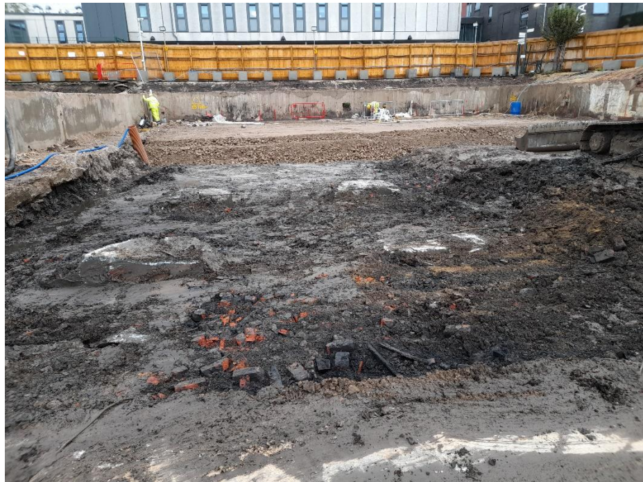
Photo 10: Ground conditions towards the centre towards the centre of the basement comprising of brick fill made ground. Photograph taken facing the north / north-east on 19/10/2021.
